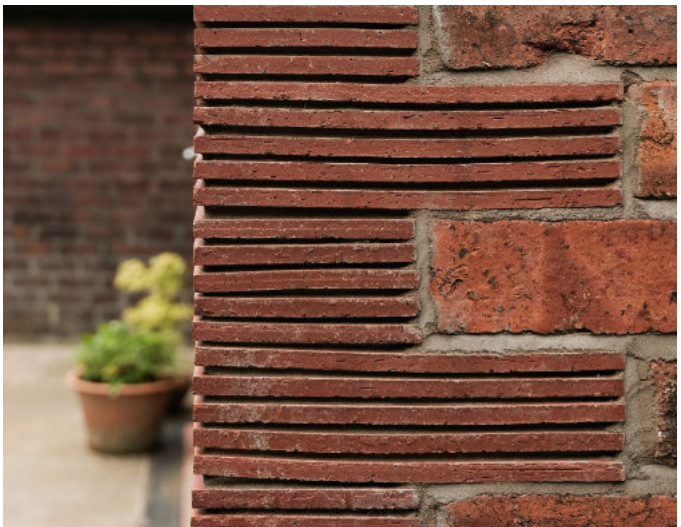
Creasing tile used as rustication.
