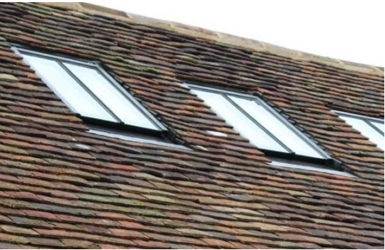
05 conservation style rooflights fit flush to tiling (black frames)
