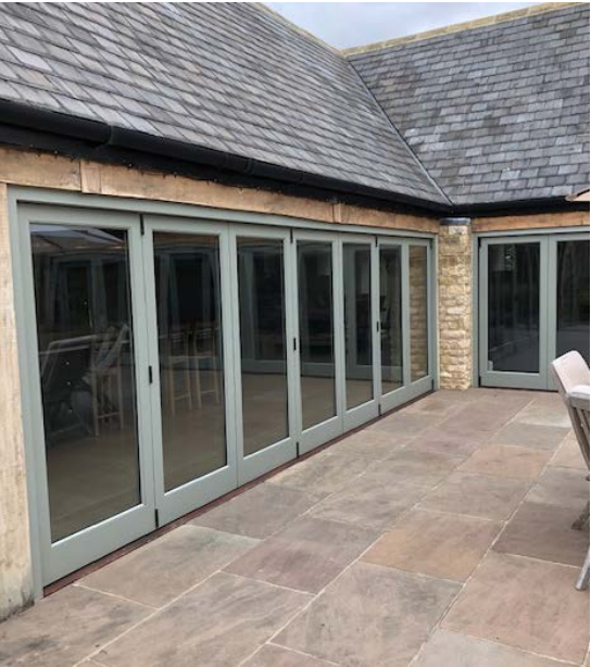
01/04 timber doors/ bifolding doors
