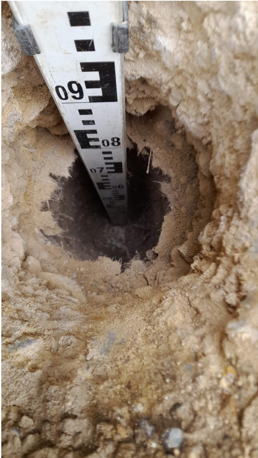
Geotextile membrane in TP03
