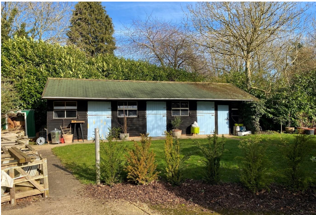
Figure 16: Stables 6. Breezeblock with timber cladding
