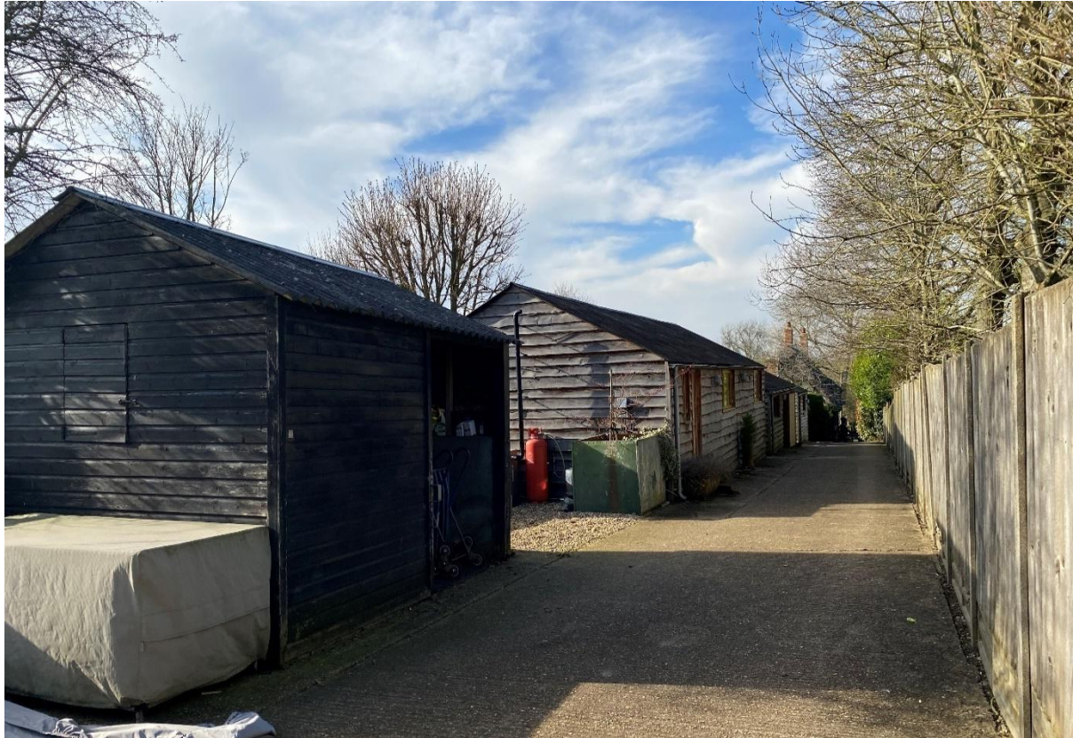
Figure 16: Timber-clad Stores 3, 4 and 5.
