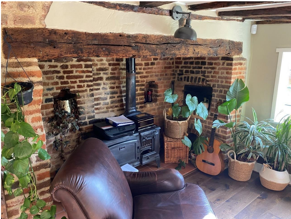
Figure 13: Fireplace range on south end of central bay, with bread oven door lined to external bread oven
