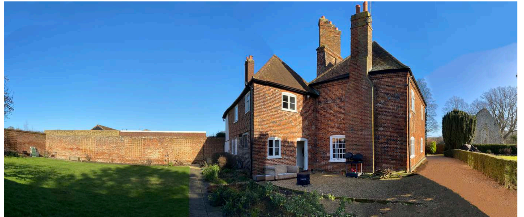
Photo-montage of south and west elevations with views of the walled garden to the west and the ruins to the east
