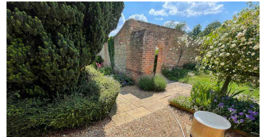
02 | northeast corner of Kitchen Garden wall
