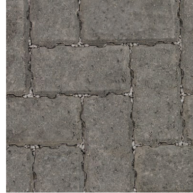
Example of permeable Block Paving 'Charcoal'
