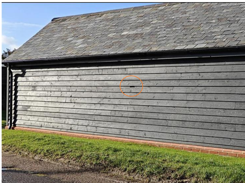
Integrated bat boxes in a timber clad building
