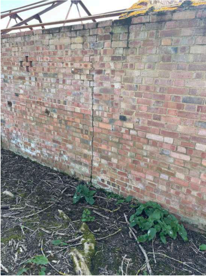
Barn 2 rear wall
