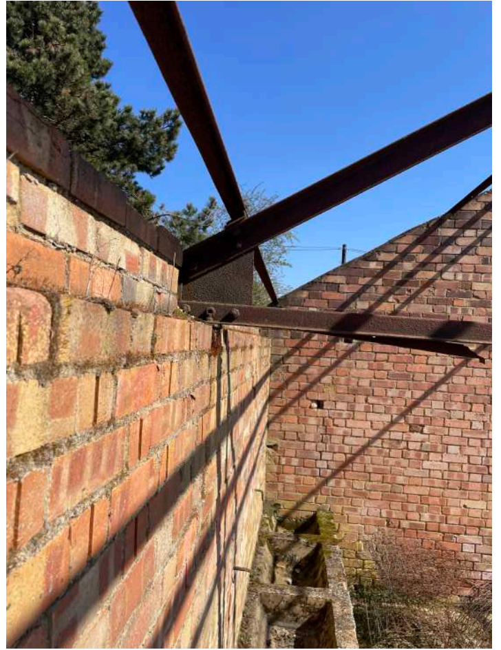
Barn 1 truss support
