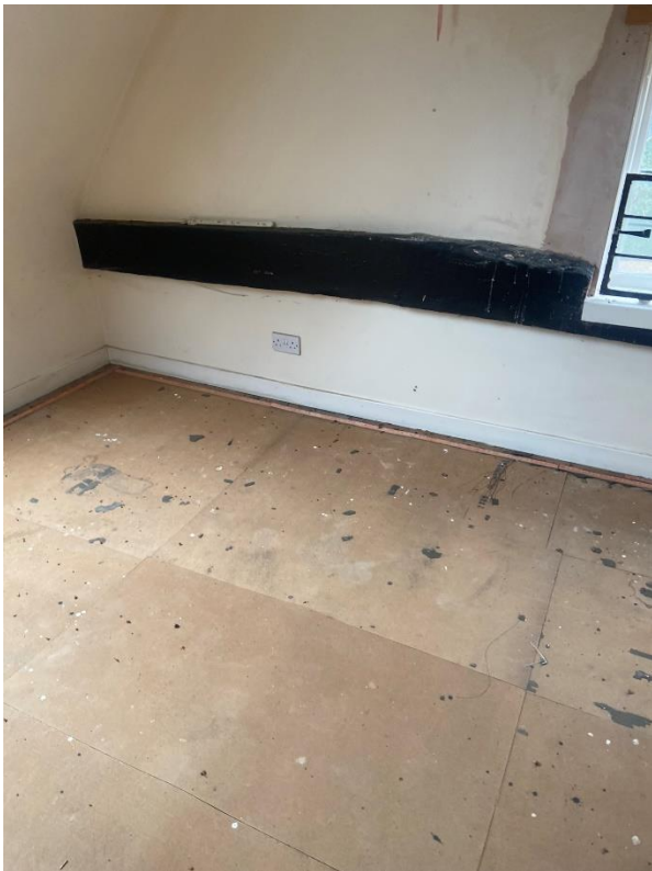
Beam in attic protrudes about 60mm will not be effected by insulation.
