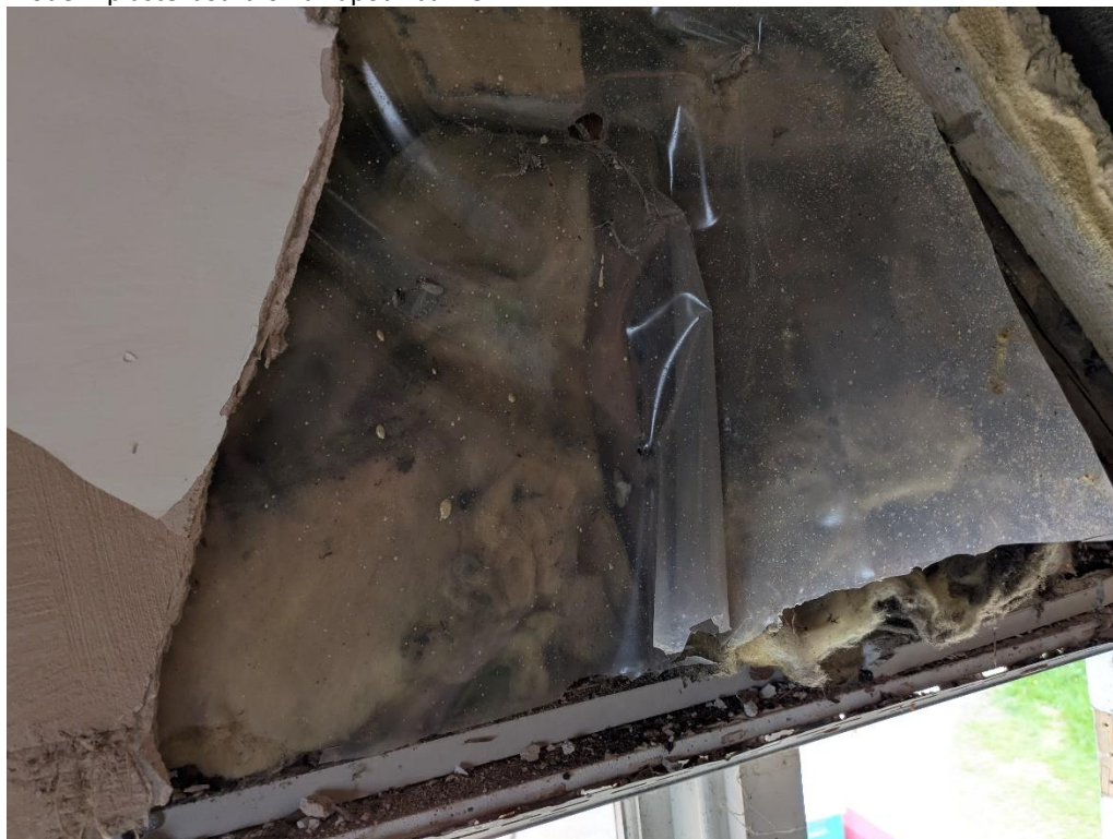
Picture of wall construction in front section of house.
