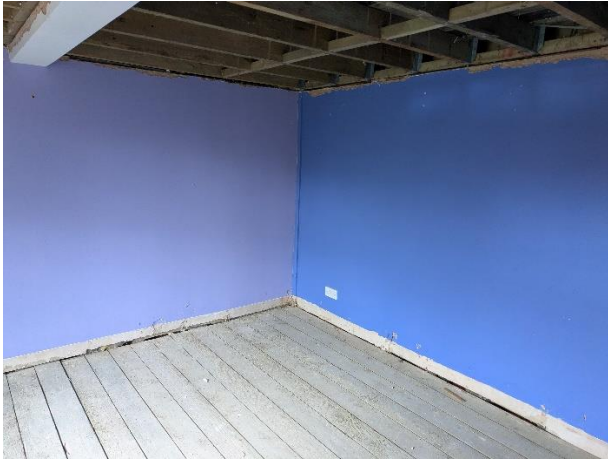
First floor room left side
