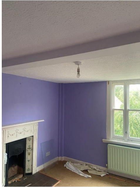
First floor room right side.
