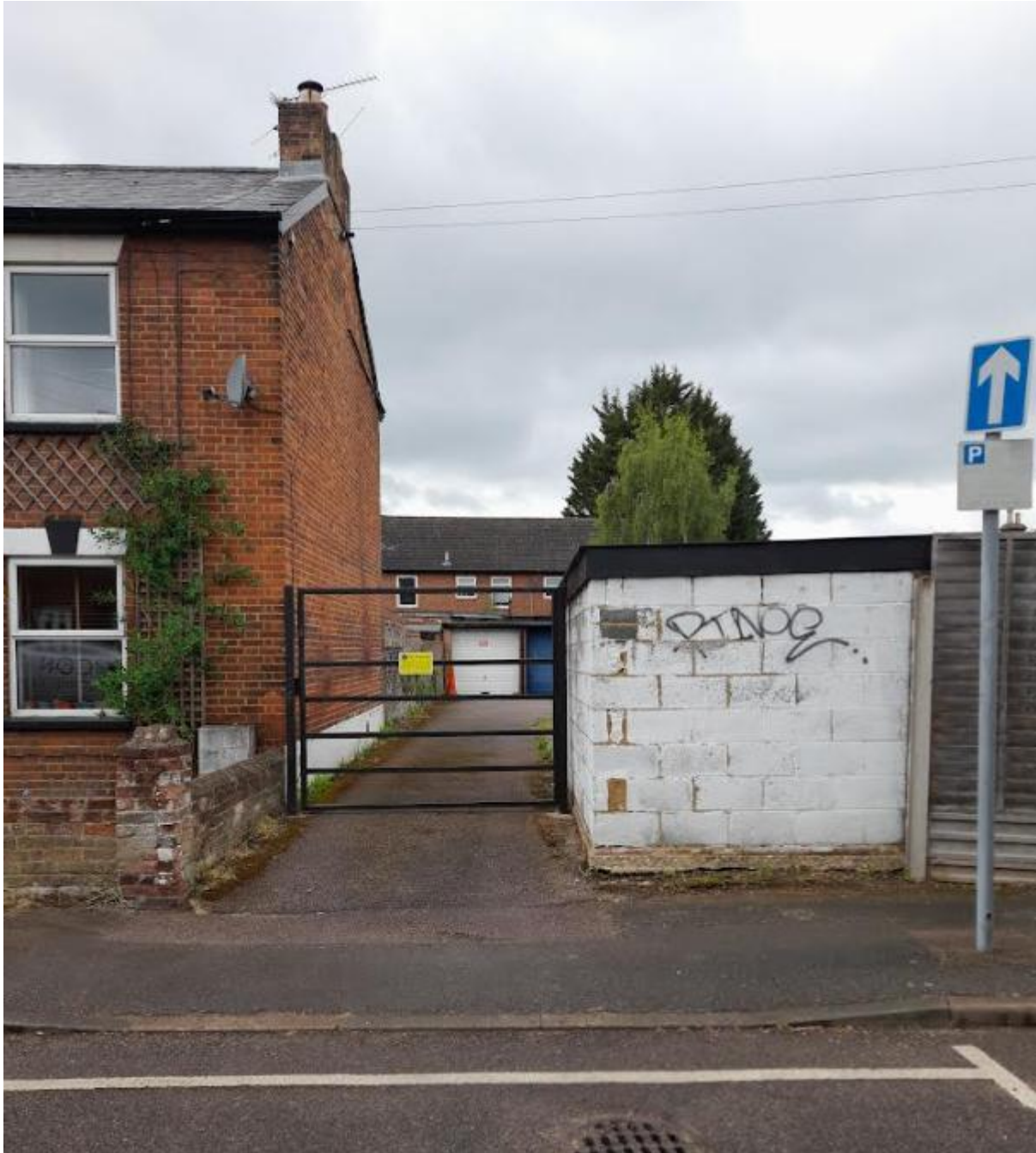
Existing vehicular access from Radcliffe Road
