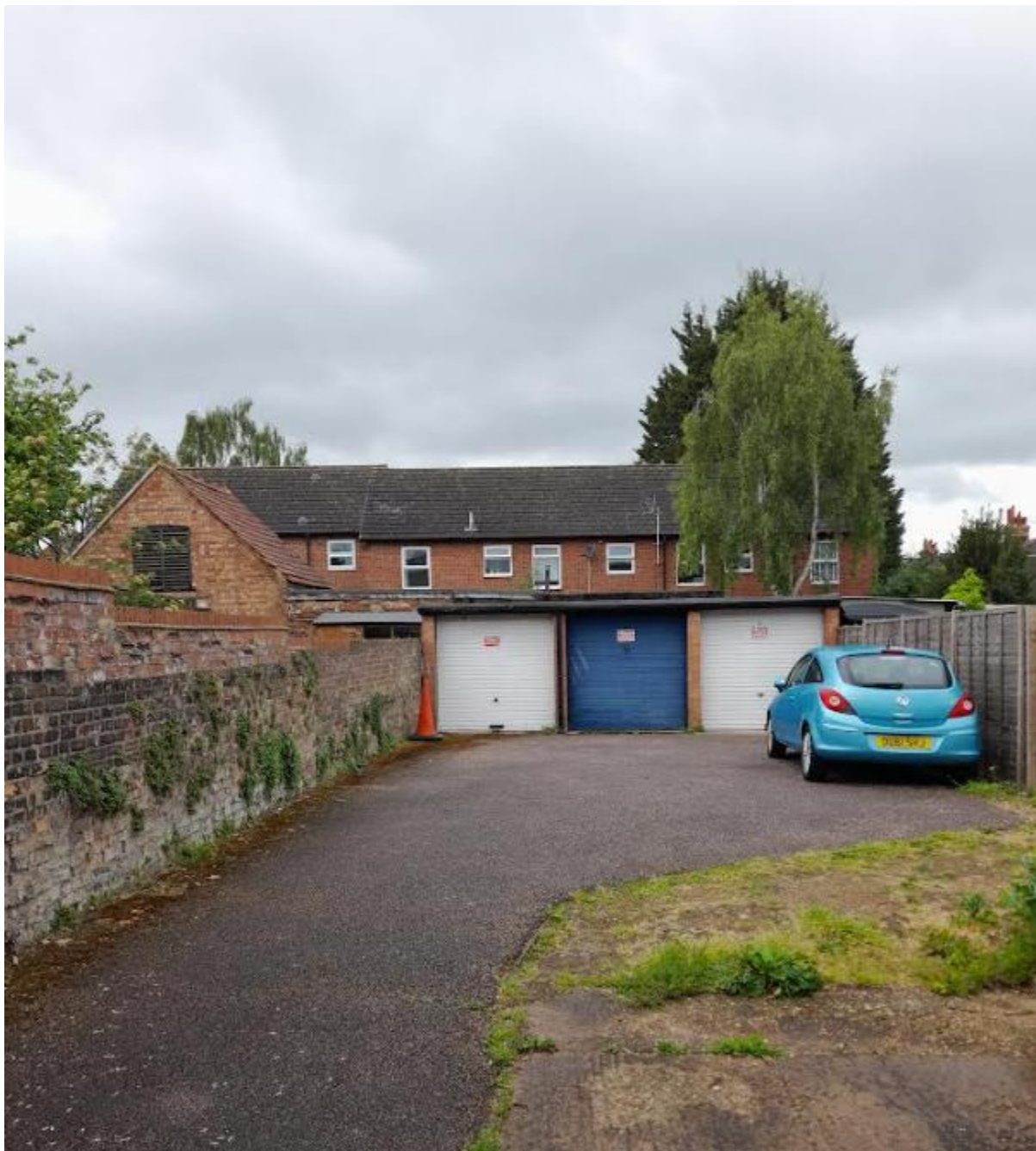
Parking courtyard off Radcliffe Road with existing building to the left of garages
