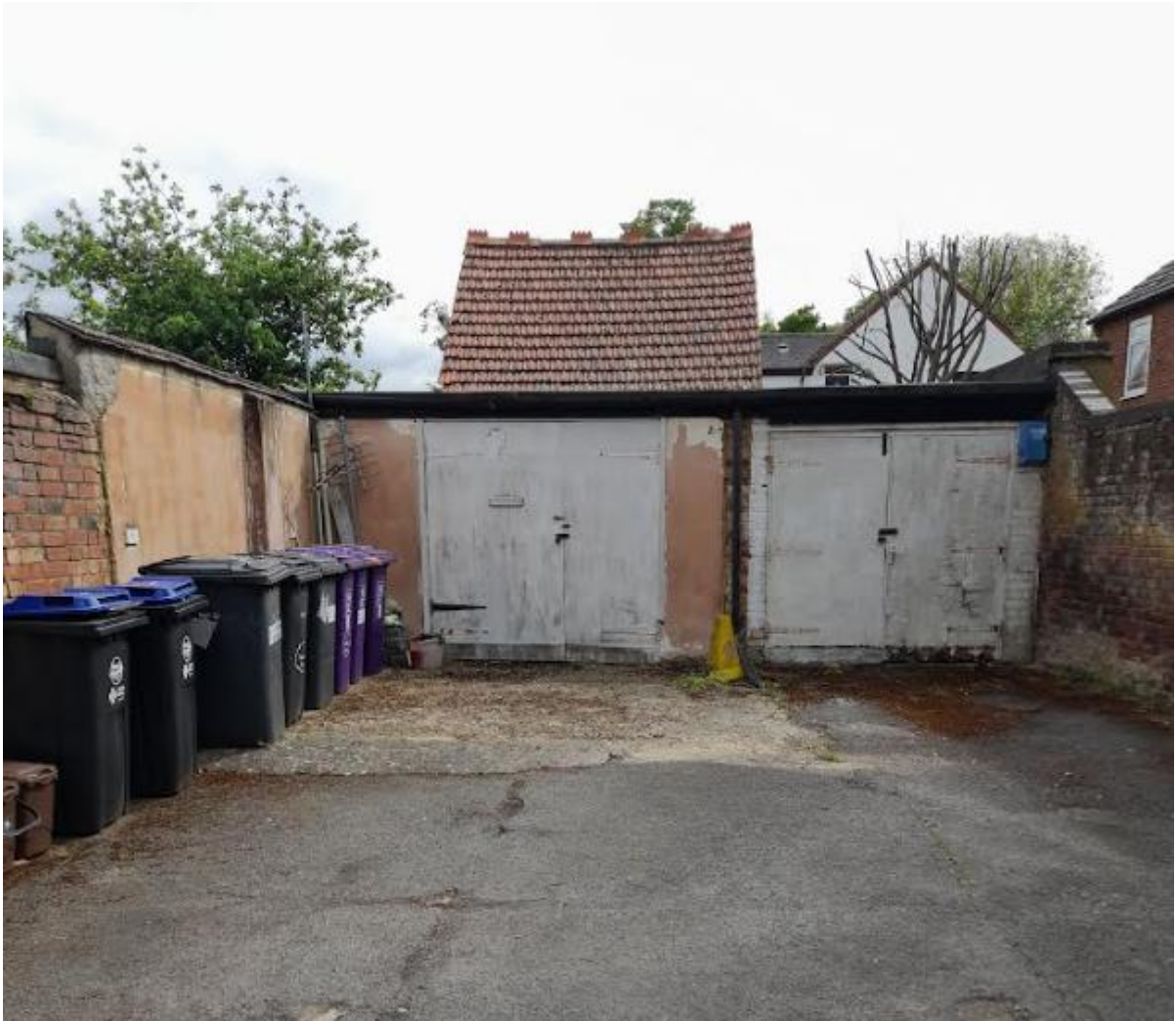
Garages and outbuilding as seen from the rear of 122 Nightingale Road
