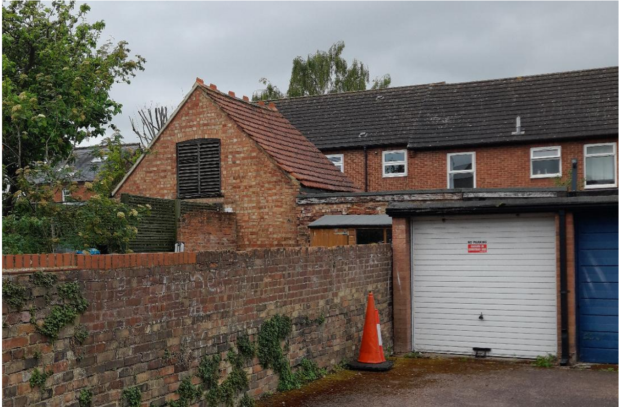
Existing former workshop building and flat roofed garages
