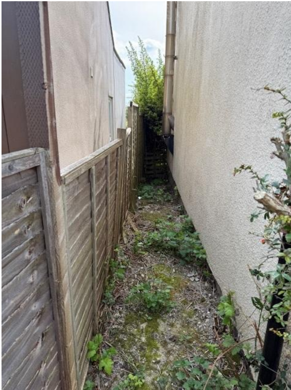
Figure 4: 5 Cambridge Road – Side passageway between 5 & 6 Cambridge Road
