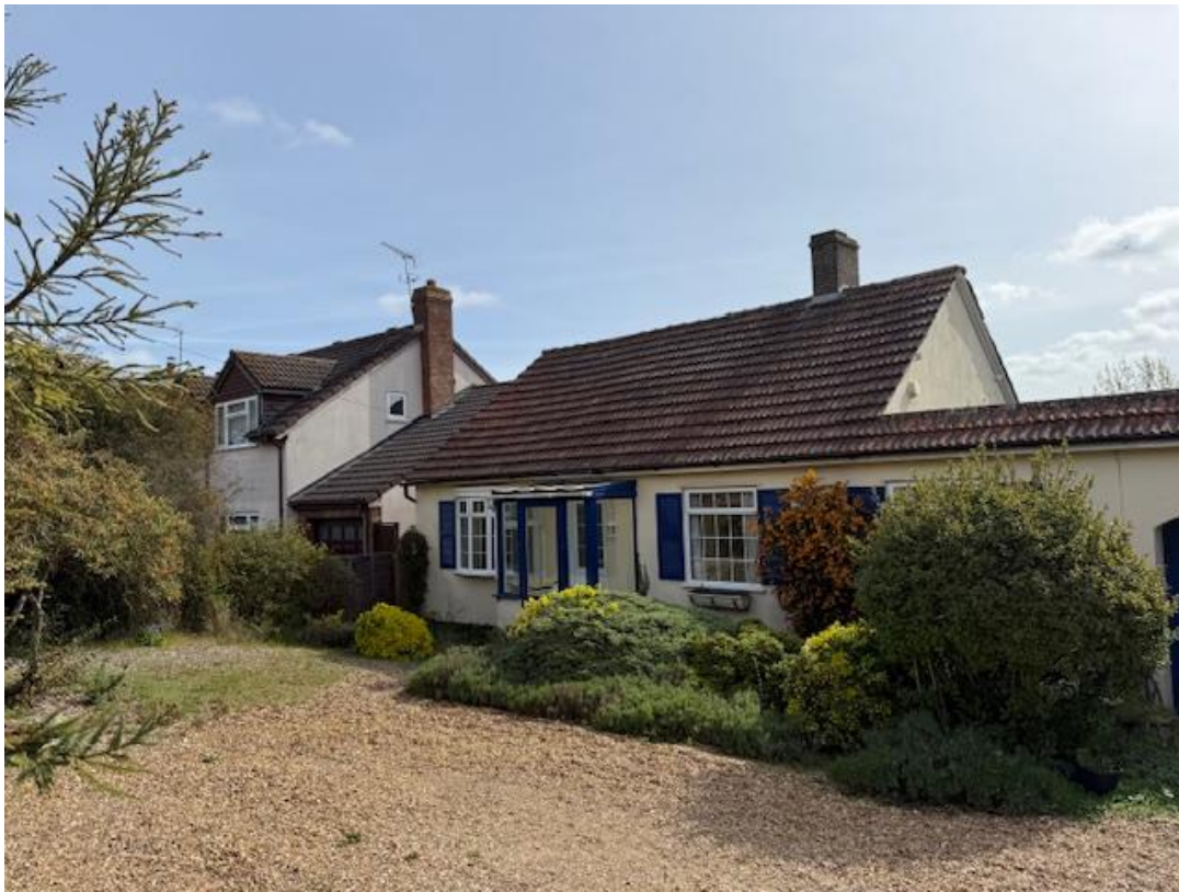
Figure 2: 5 Cambridge Road - Front Elevation & 6 Cambridge Road
