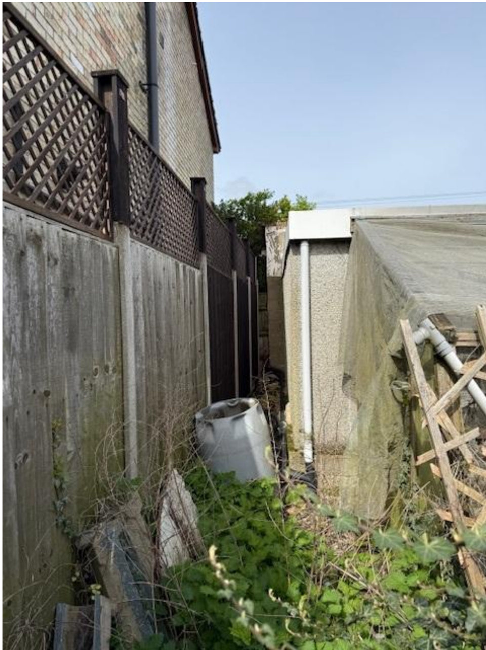
Figure 15: 5 Cambridge Road – Space between 4 & 5 Cambridge Road
