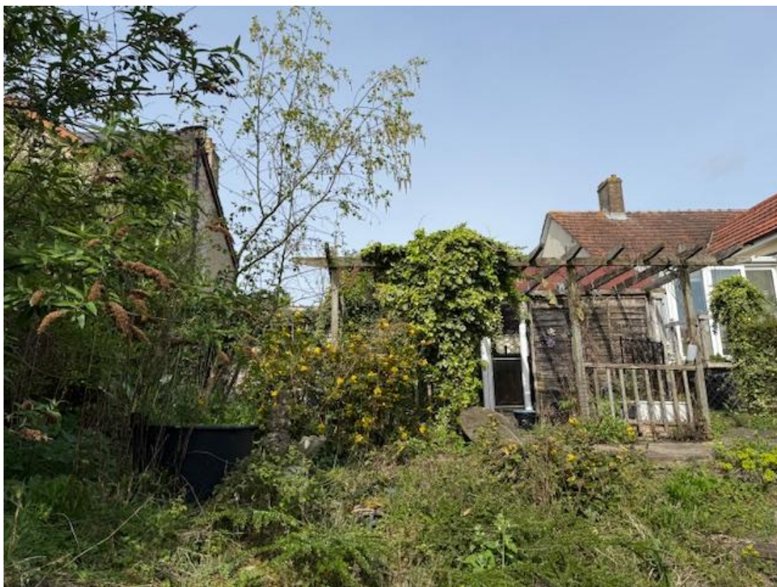
Figure 11: 5 Cambridge Road – Outbuilding & side of 4 Cambridge Road
