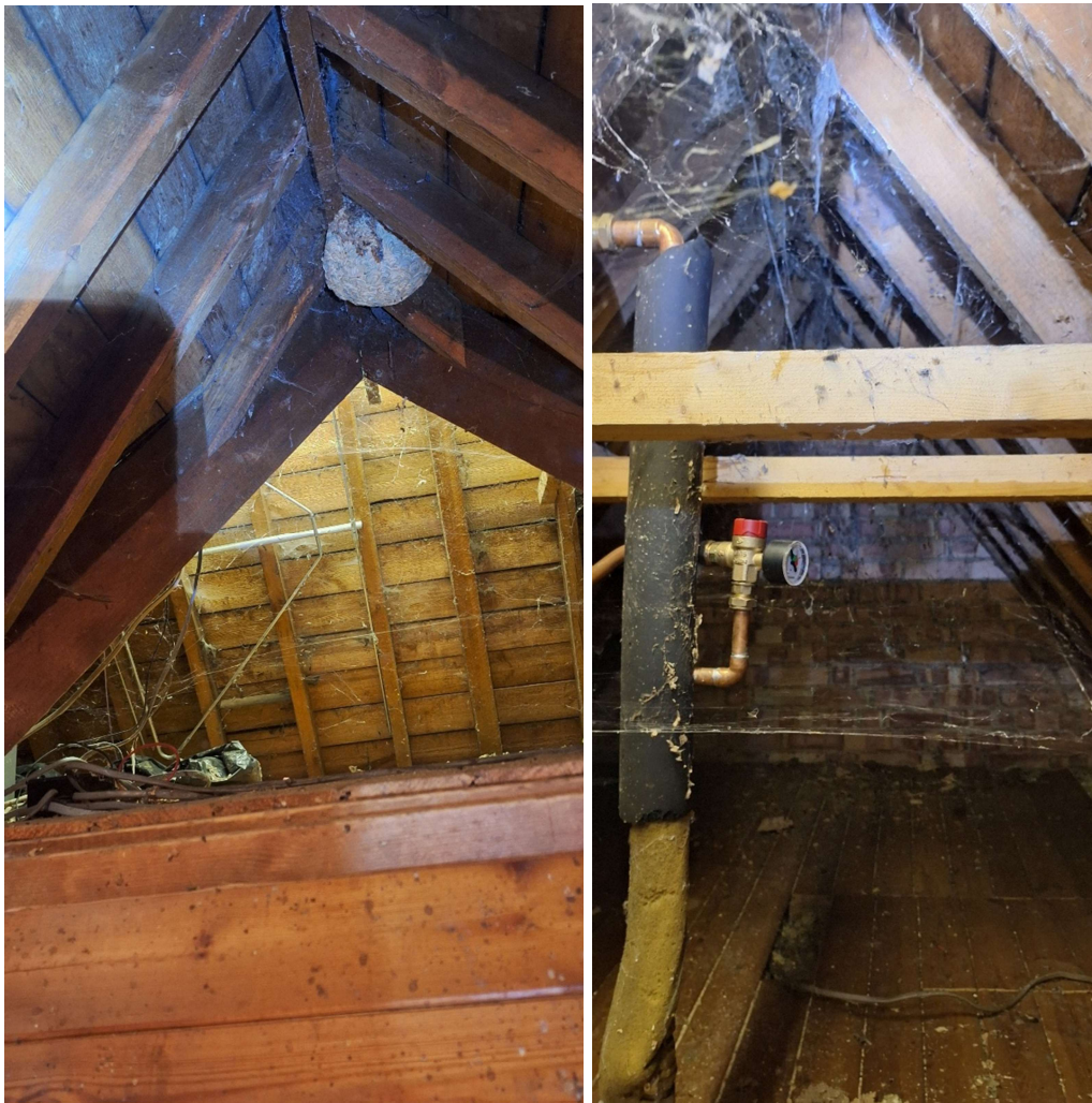
Photographs 3 & 4. Interior of loft space, Building A. Note webs, wasp nest and good state of repair.
