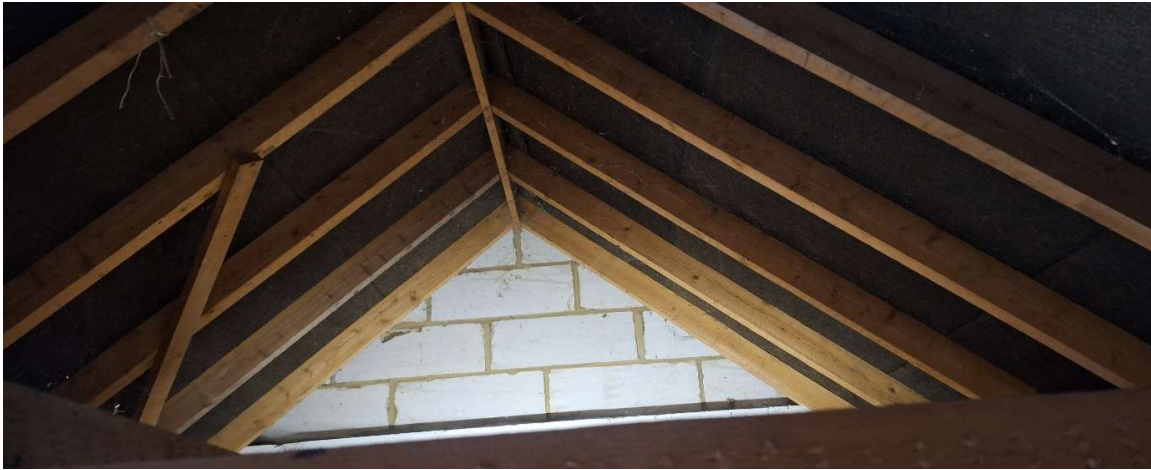
Photograph 5: Interior of the roof space, Building B
