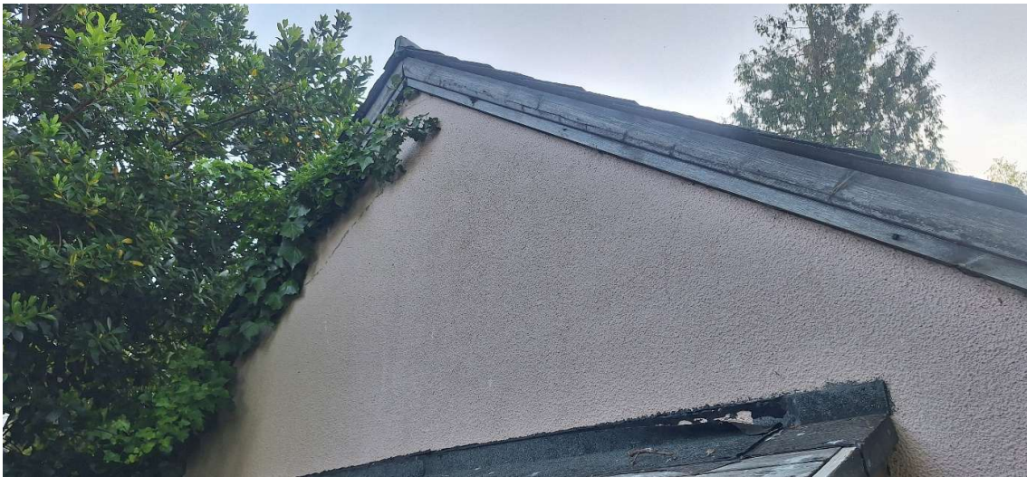
Photographs 13&14. Rendering and eaves with negligible roost potential, Building A
