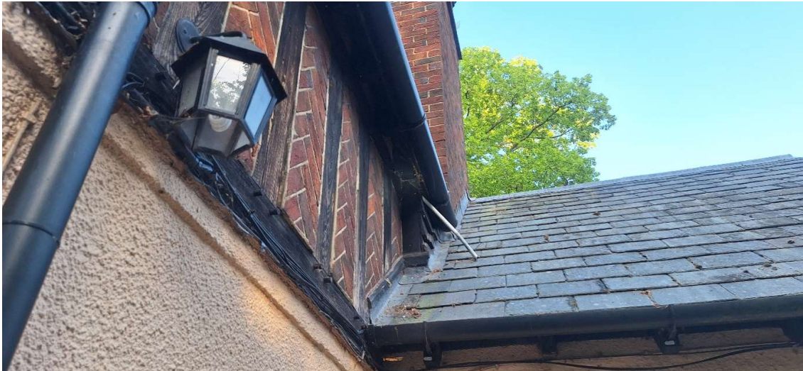
Photograph 2. Building B showing herringbone brickwork, lead flashing, slate tiles and render. Note overall good repair.
