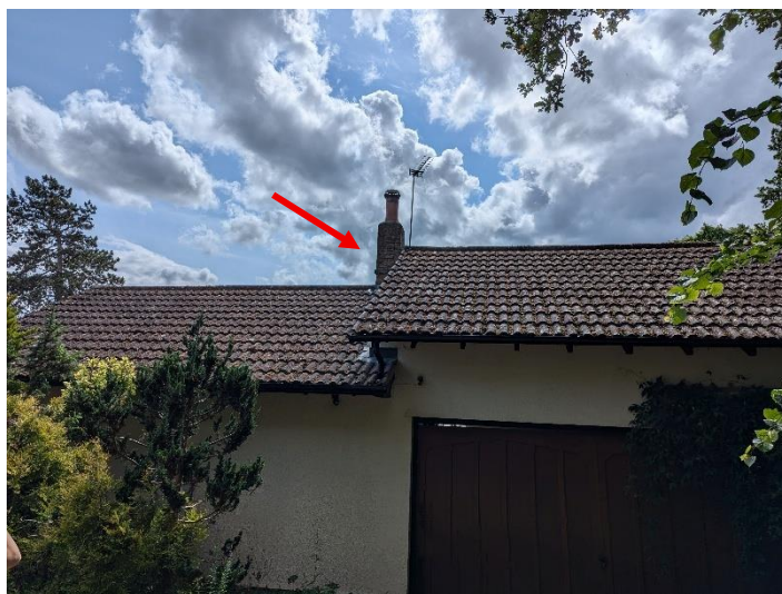
Figure 3: Northeast elevation of garage (right) and adjoining room. Arrow depicts location of feature identified in Figure 4
