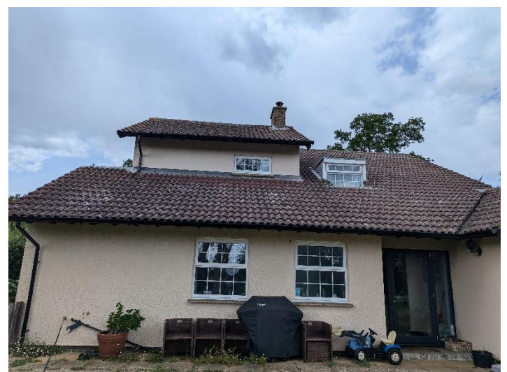
Figure 10: Northwest elevation of central building
