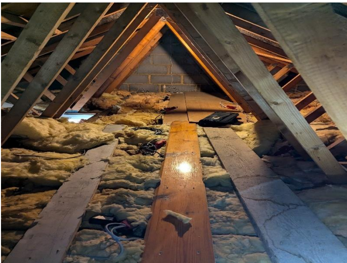
Figure 13: Loft space above single storey
