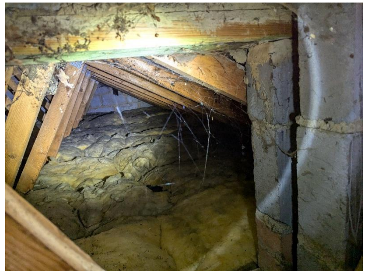
Figure 14: Loft space above two-storey
