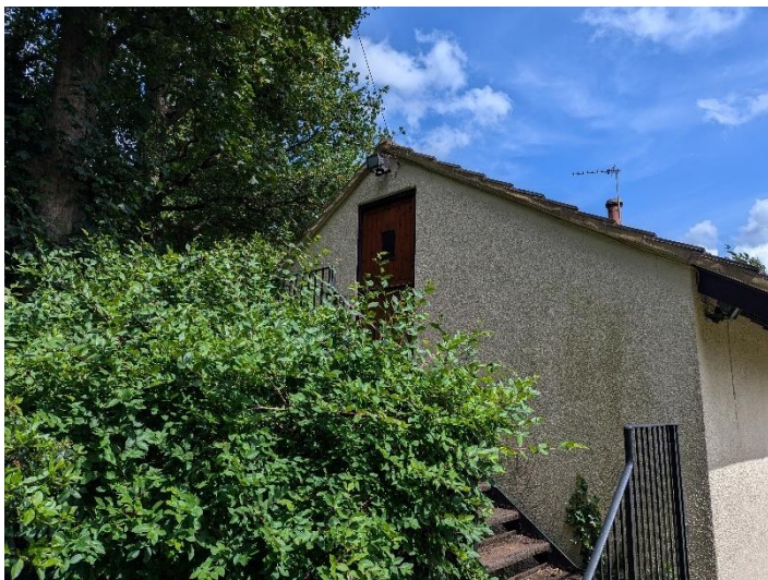
Figure 7: Northwest gable end of garage
