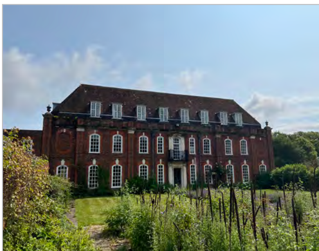
Photo 3 - West Wing west facade
