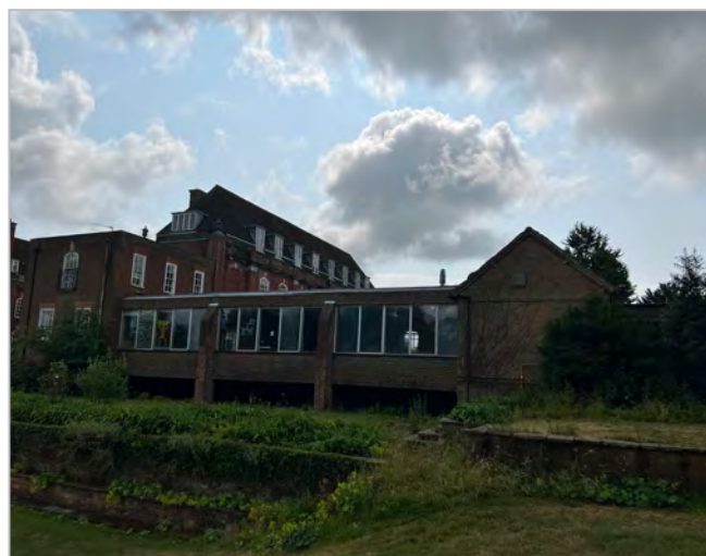
Photo 4 - West Wing (back) and West Spur
