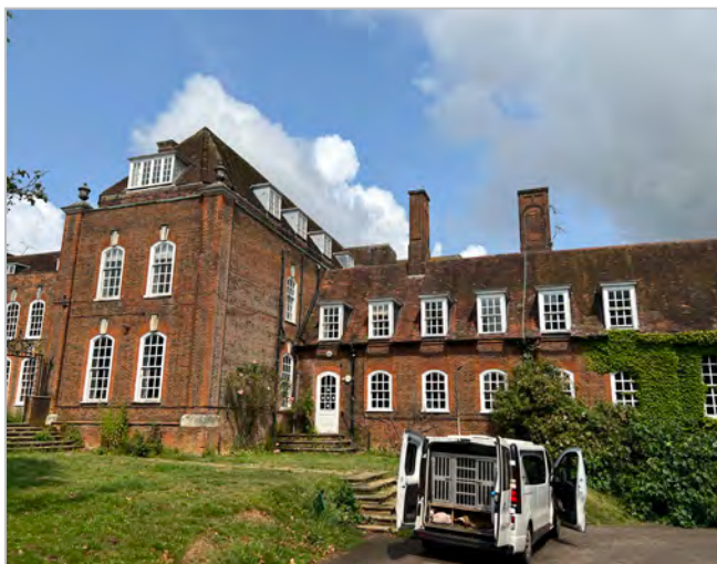
Photo 1: Old House & East Wing - north facade
