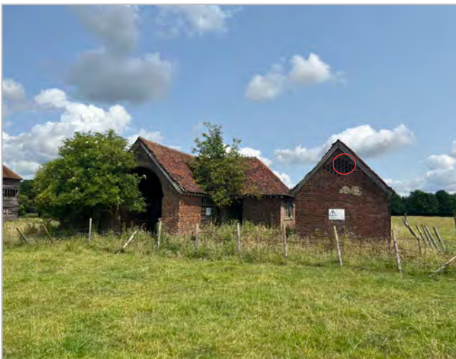
Photo 11 - Pumping station. Roost exit point circled
