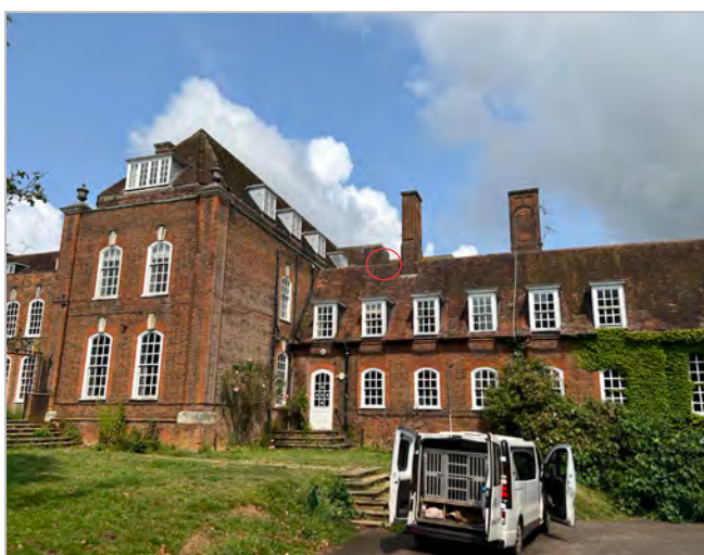
Photo 5 - East Wing & East Annex. Bat roost location on East Annex circled
