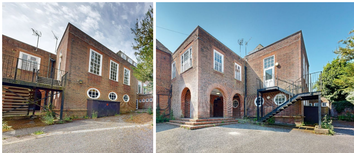
Present day photos of the rear elevation of east block (dated 2023)
