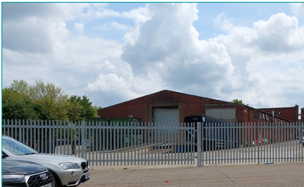
Figure 3 - Photo of yard area (looking towards 5 Hunting Gate building) which is fenced and gated at the rear with access primarily from Hunting Gate.
