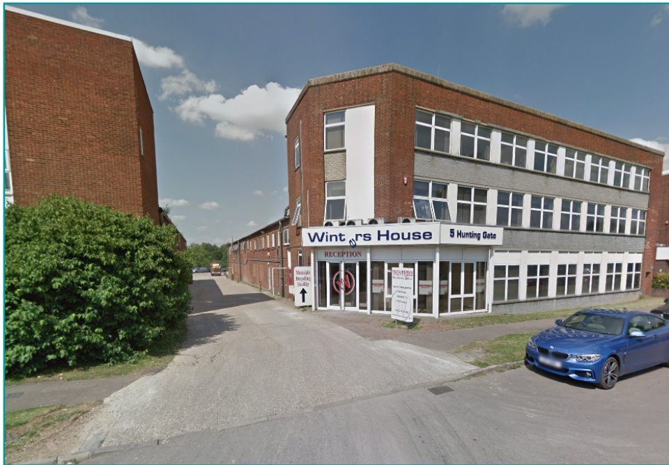
Figure 2 - Google Image of the Site from March 2019 showing front office area.
