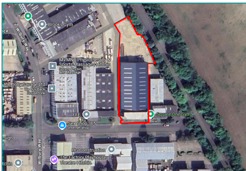
Figure 1 - Google Earth Image of the Site from June 2023 - Site indicated in red.
