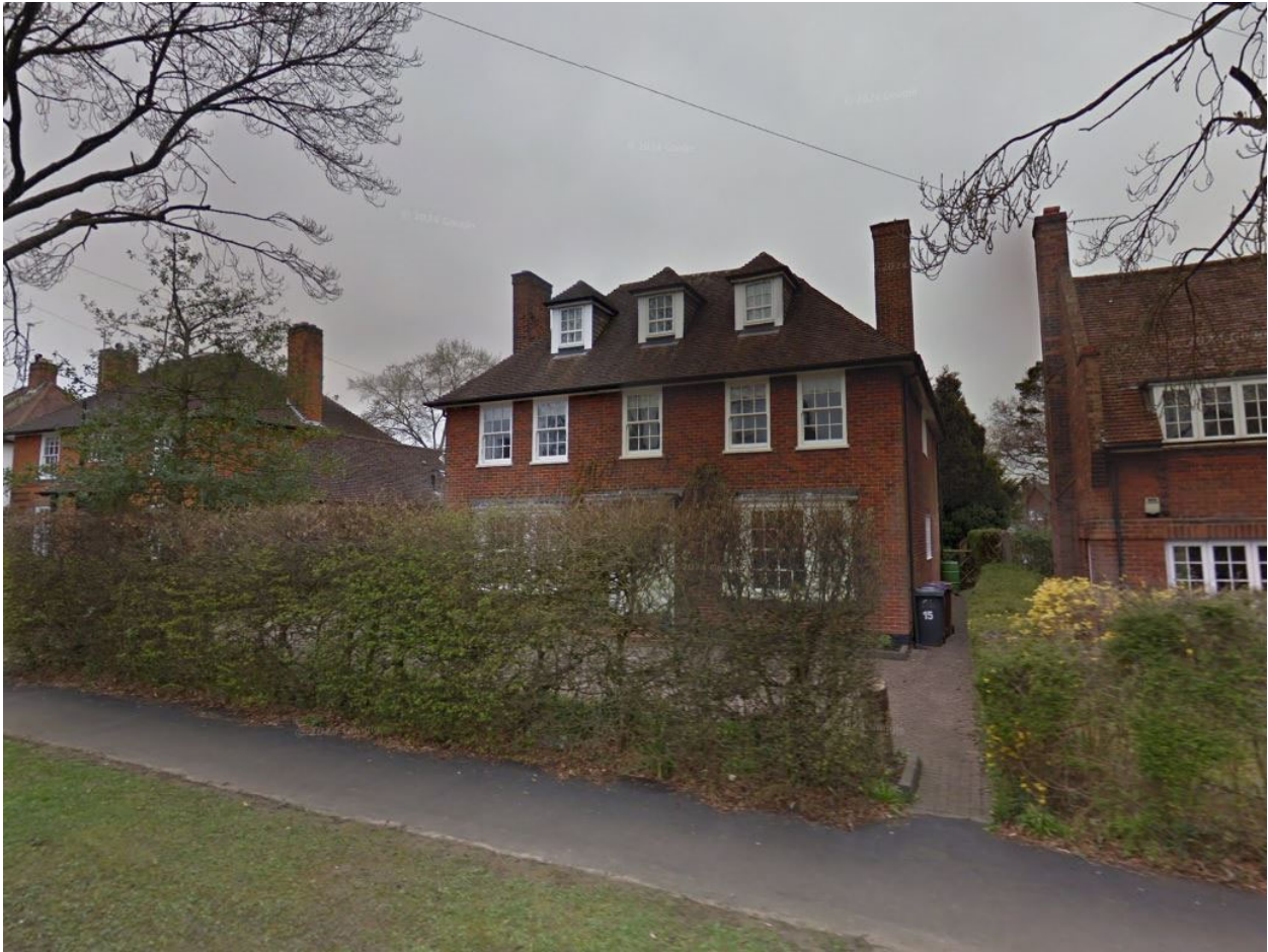
ABOVE: Image of no.15 to the north, built in an identical style but featuring 3no. dormer windows to the front elevation. Image © Google
