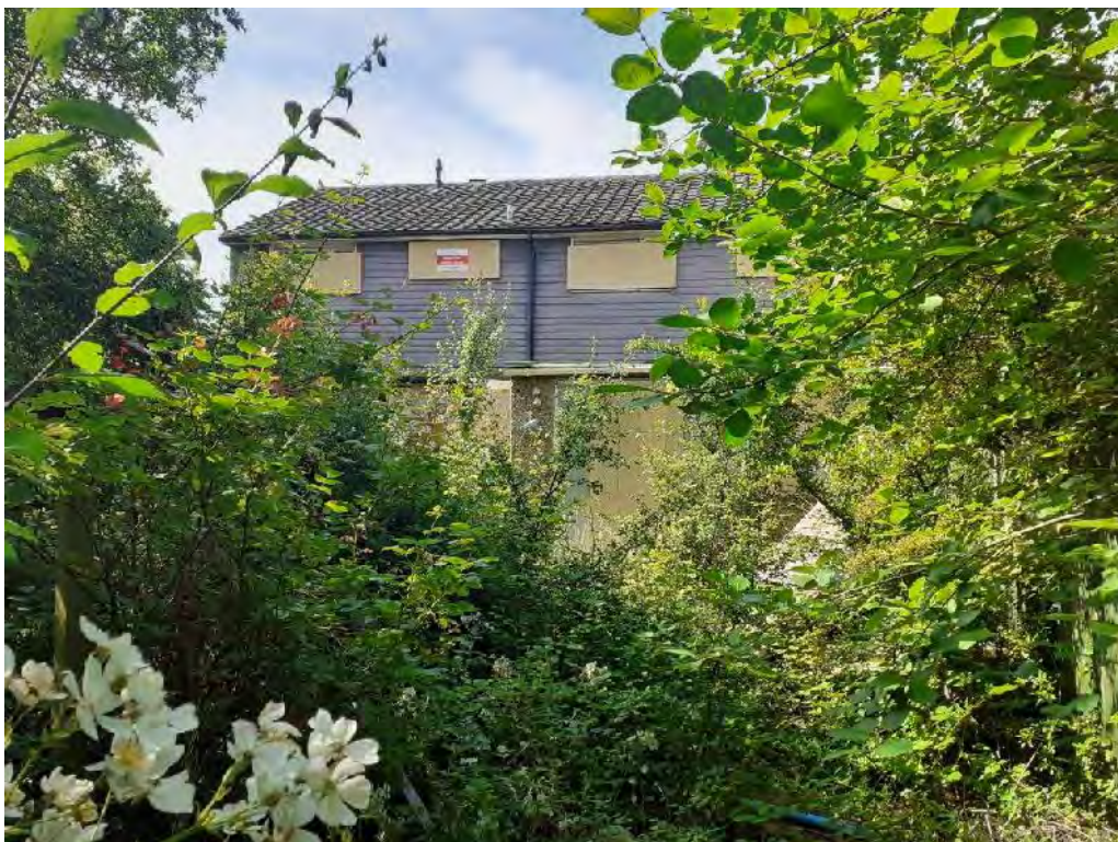
Plate 6: Rear garden of No. 3 Newells, which is overgrown and derelict, taken from the north.
