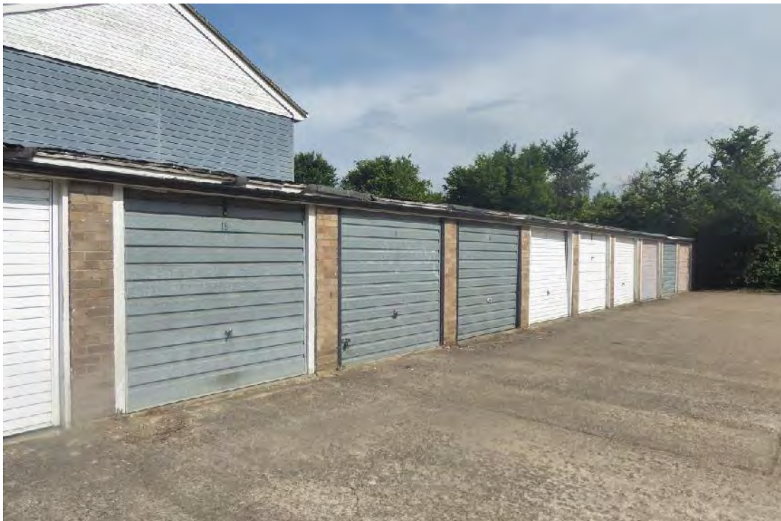
Plate 8: Westernmost row of ten single storey modern garages located in the western section of the Site, taken from the south-east.
