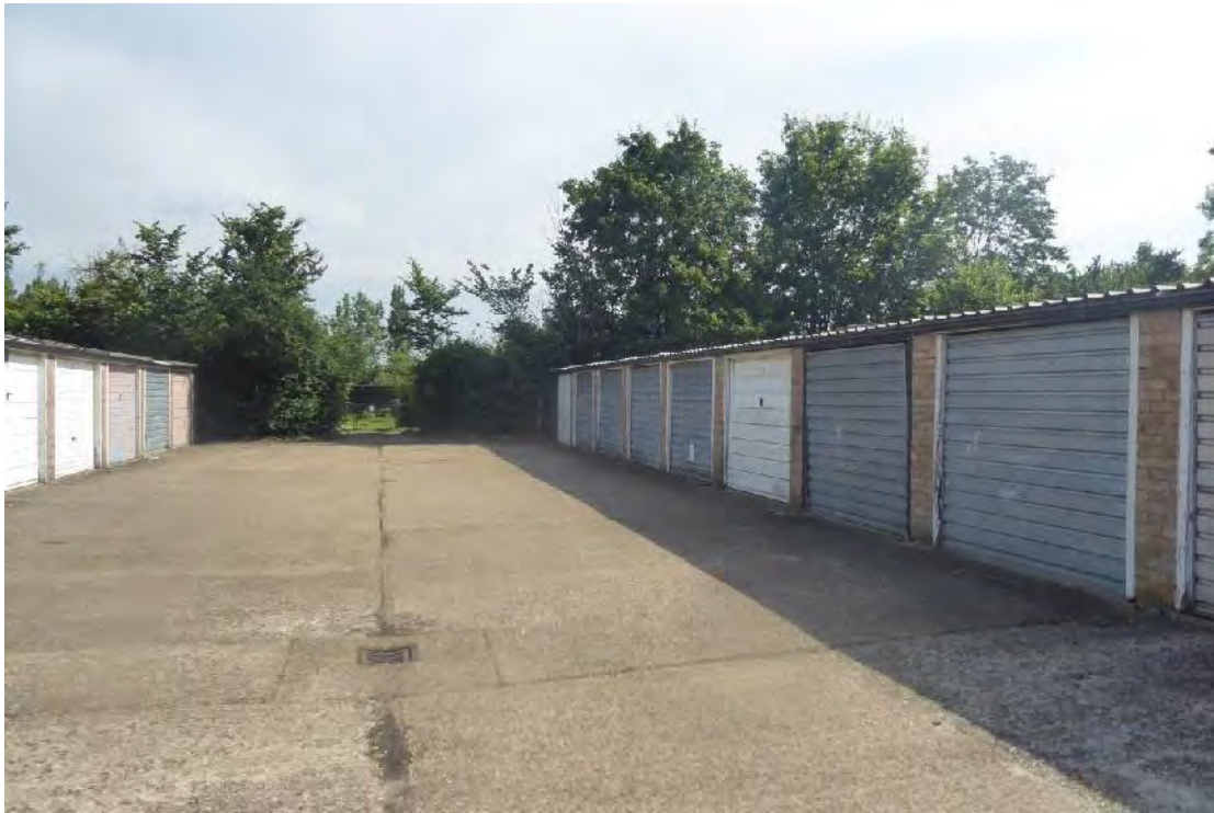
Plate 7: Two rows of ten single storey modern garages located in the western section of the Site, taken from the south.
