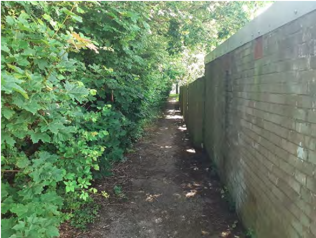
Plate 13: Hardstanding pathway located to the immediate north of the Site and which provides access to the rear gardens of Nos. 3 – 5 Newells, taken from the west.
