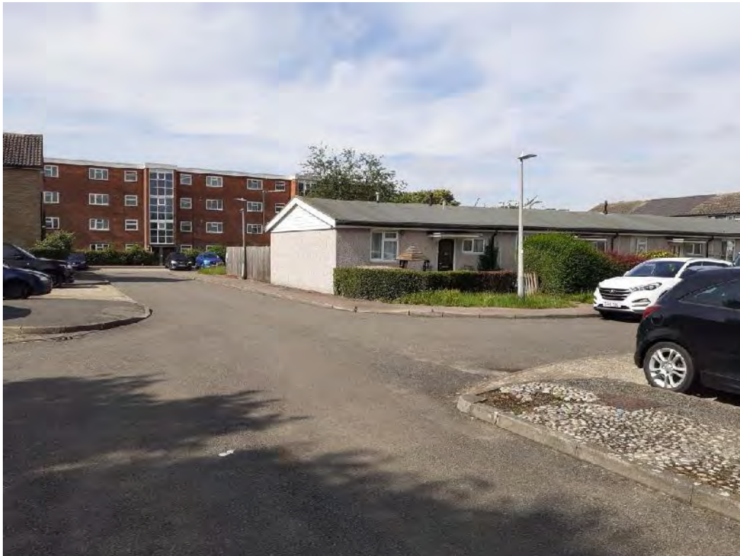
Plate 11: Course of the metalled road of Newells located in the southern section of the Site, taken from the north-west.
