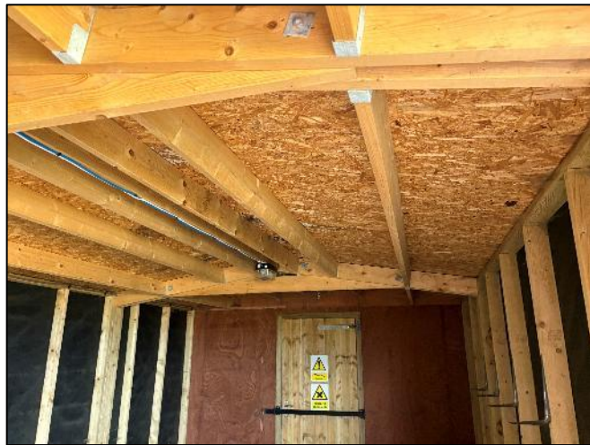
Photograph 5 Interior of shed
