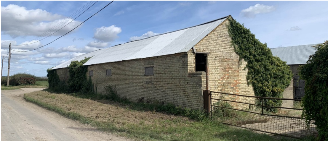
Figure 6. West elevation of west wing
