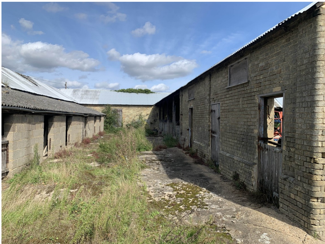
Figure 10. West elevation of east wing and south elevation of north wing
