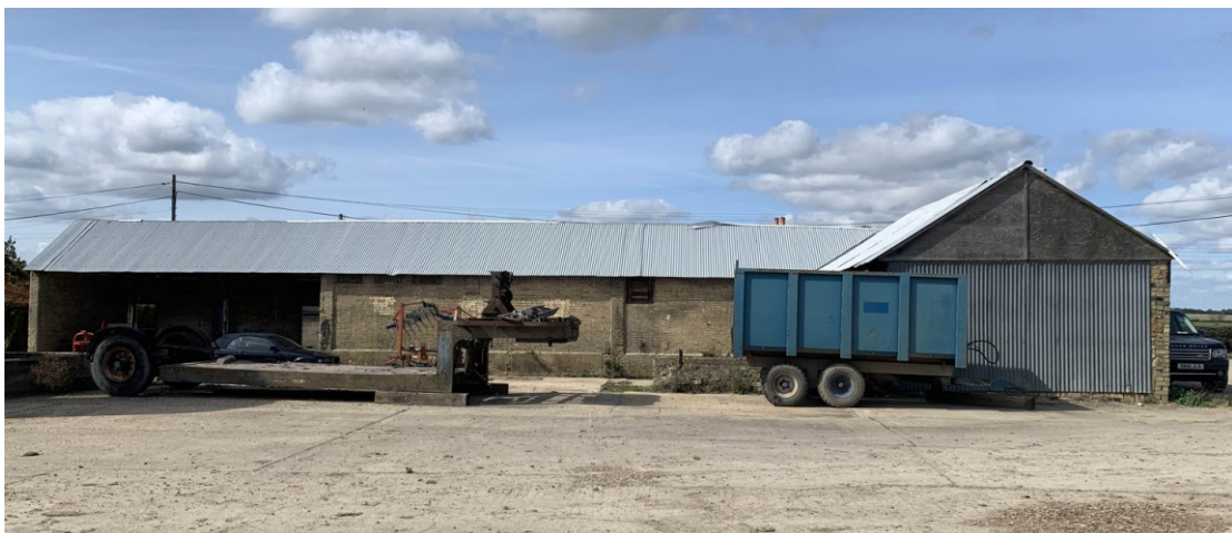
Figure 8. East elevation of east wing
