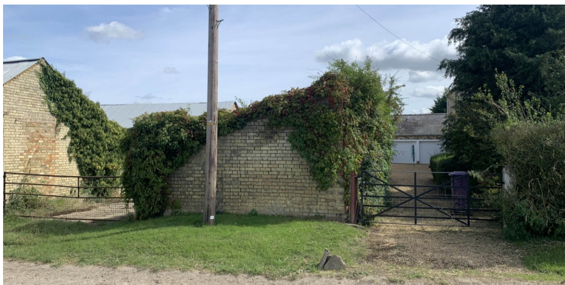
Figure 12. West elevation (Northfield Road)
