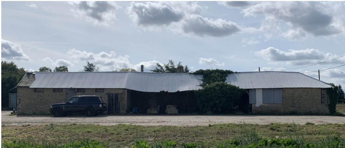
Figure 7. North elevation of north wing
