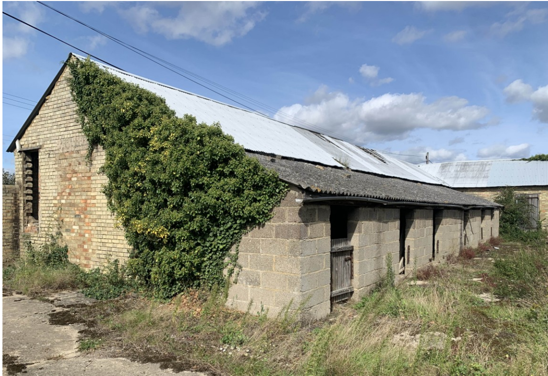
Figure 9. South and east elevations of west wing
