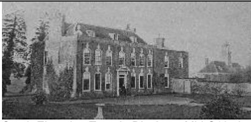
South Elevation Temple Dinsley – Mid C19 shows the Georgian front of Temple Dinsley prior to any wing to the West. One of the earliest photographs. Outbuildings to the West are not visible we know from the early historic maps that these buildings existed.
