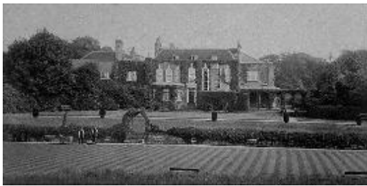
North Elevation. Photo taken prior to the Lutyens' 1909 West Wing.
