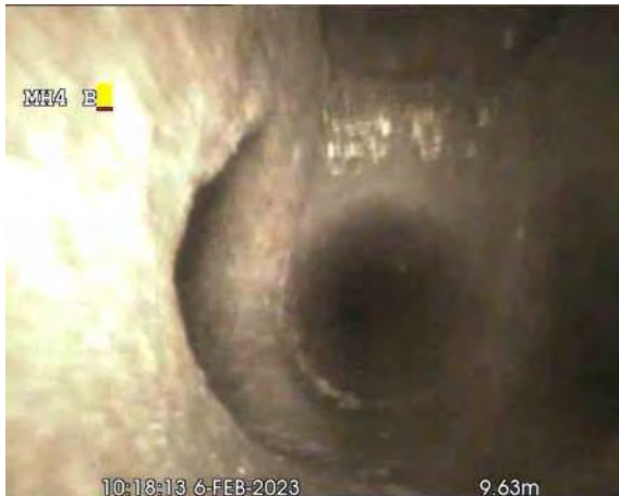
1aa8beed-8b10-4fb9-bd2a-54018b71e46a.jpg, 00:00:38, 9.83 m Junction at 3 o'clock, 100mm dia
