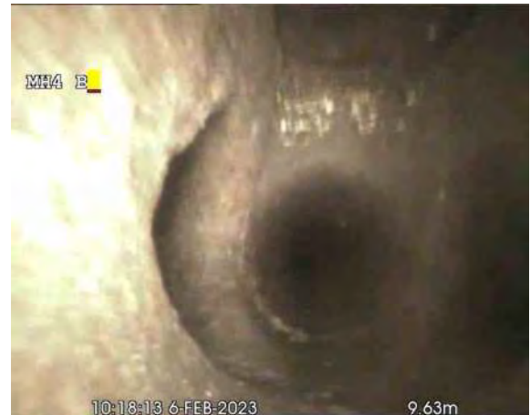
ee64899a-ccf0-4f8f-aebf-3013d63588b8.jpg, 00:00:38, 9.83 m Junction at 9 o'clock, 100mm dia
