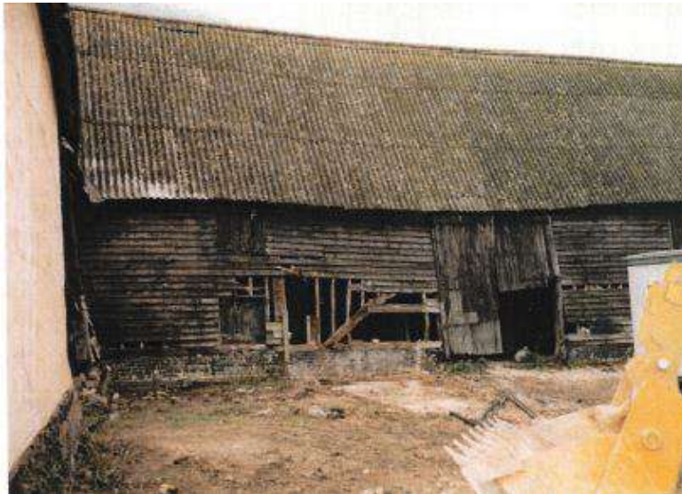
Daubentons Barn in the early stages of the building work to convert it to residential in the 1990's
