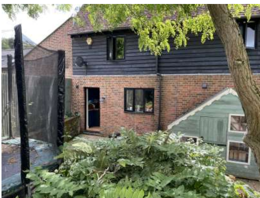
Rear elevation of Daubentons Barn showing the non-historic cavity masonry wall up to first floor level.
