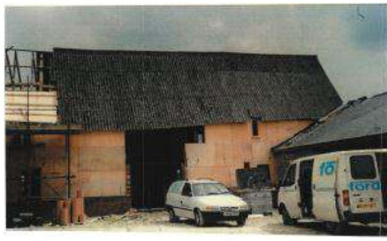
Daubentons Barn with the timber frame bracing being added and openings appearing.
