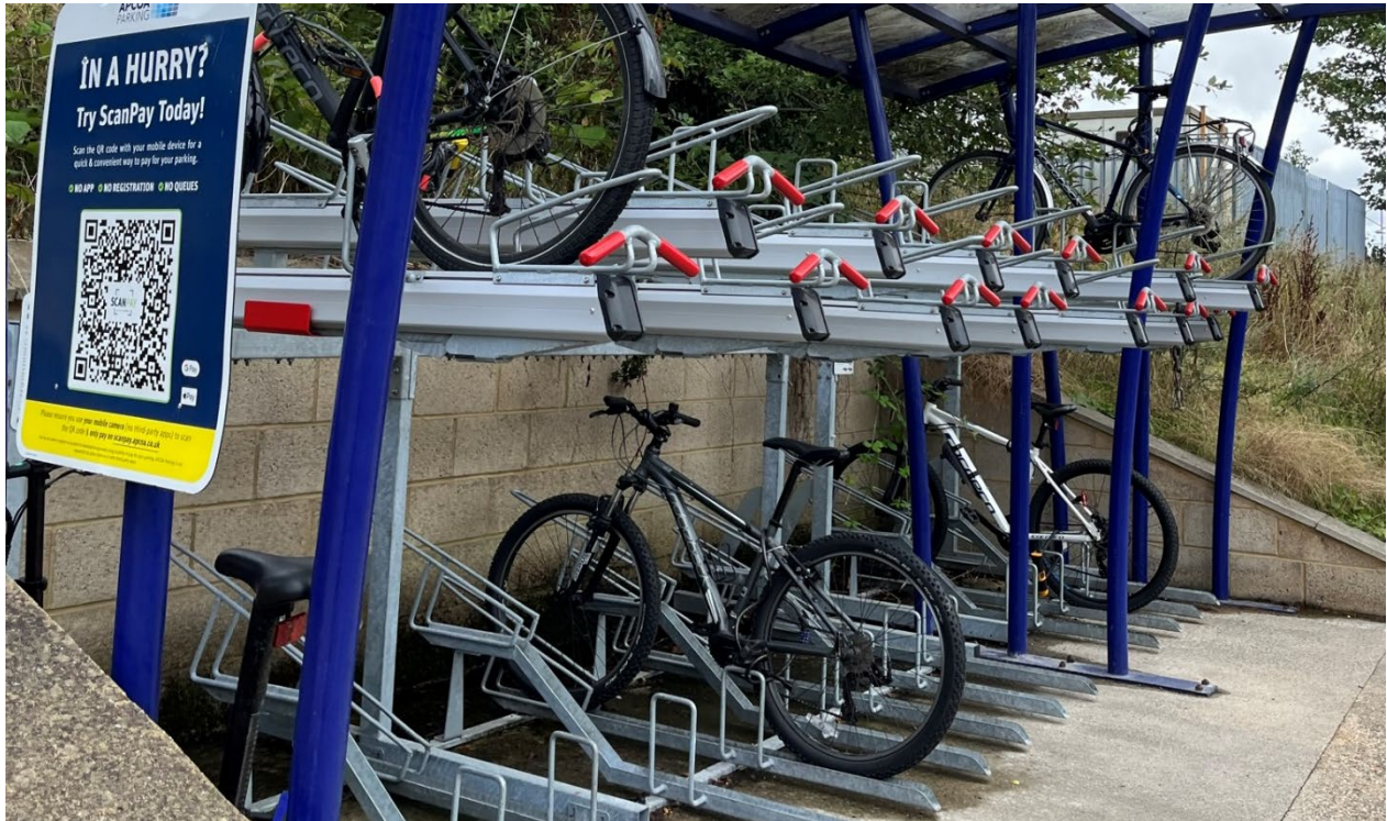
Figure 2-7: Cycle Parking At Baldock Railway Station
