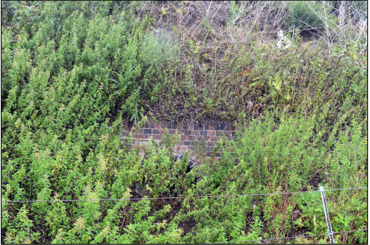
Plate 21: Drain or tunnel under the railway at the north of BA10, looking north-west
