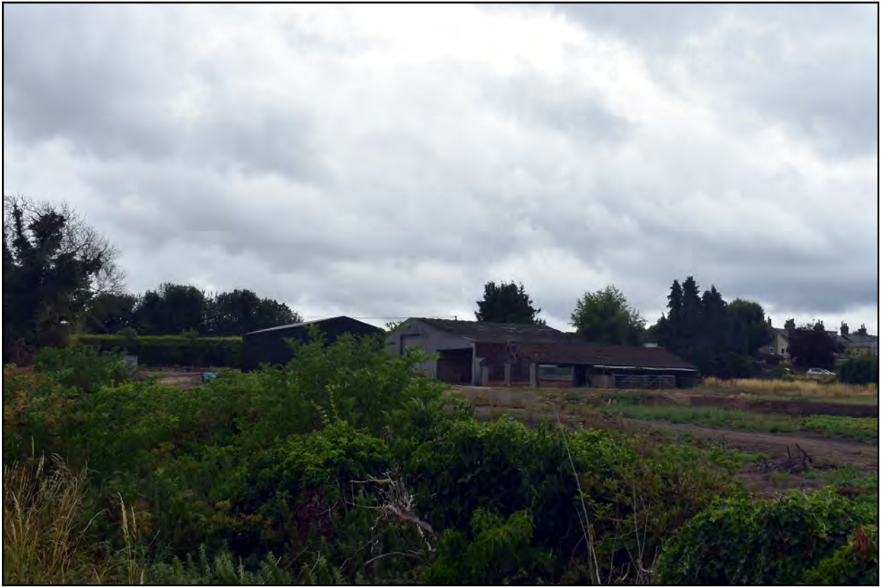
Plate 3: Barns in the south-west of BA1, looking south-west
