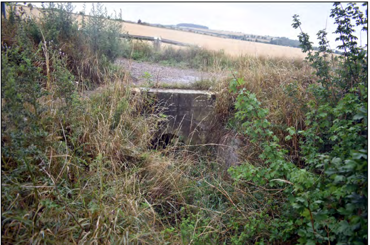
Plate 18: Drain across BA3, looking south
