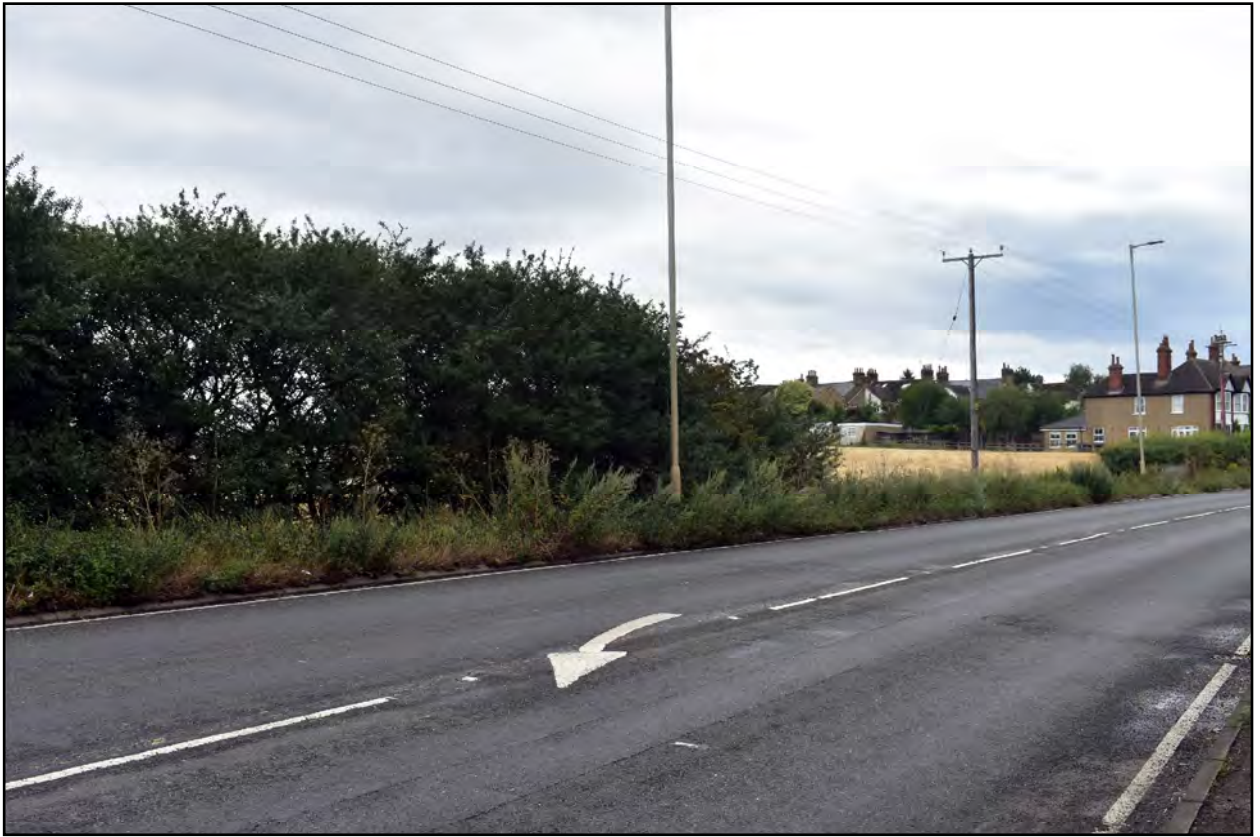
Plate 5: Overhead cables and street lights along the western edge of BA1, looking south-east
