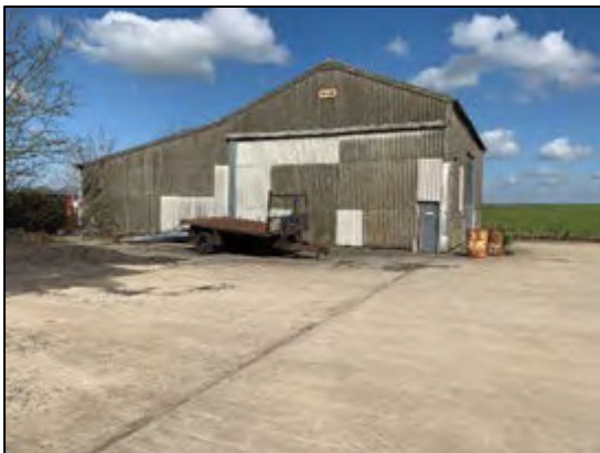
Photograph 5: example of buildings and hard standing within the Site
