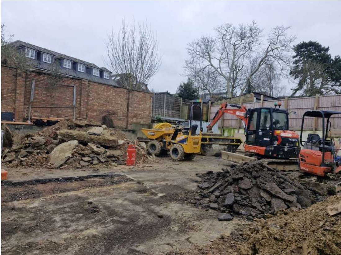
Photo 1: Showing SEC conducting a Watching Brief during removal of Tarmac and Concrete hardstanding.
