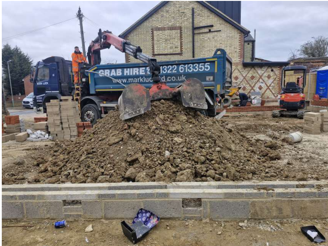
Photo 5: Showing the removal of more waste arisings.
