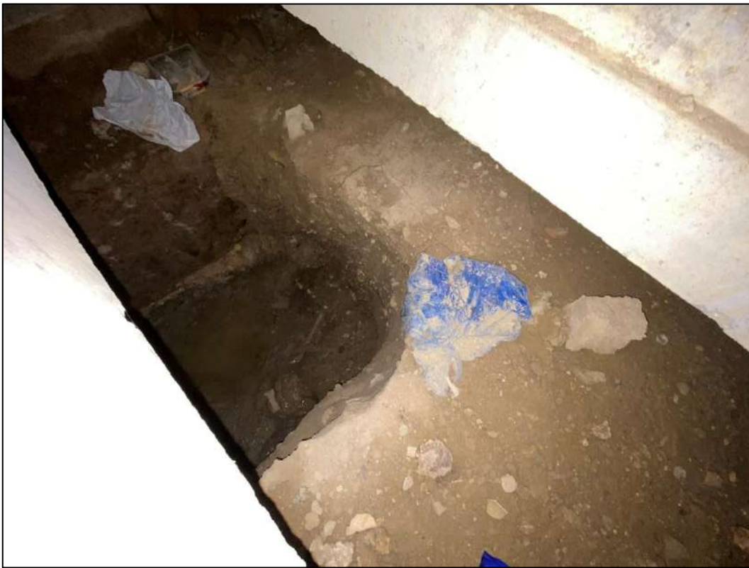
Figure 3-A: Excavation under building footprint
