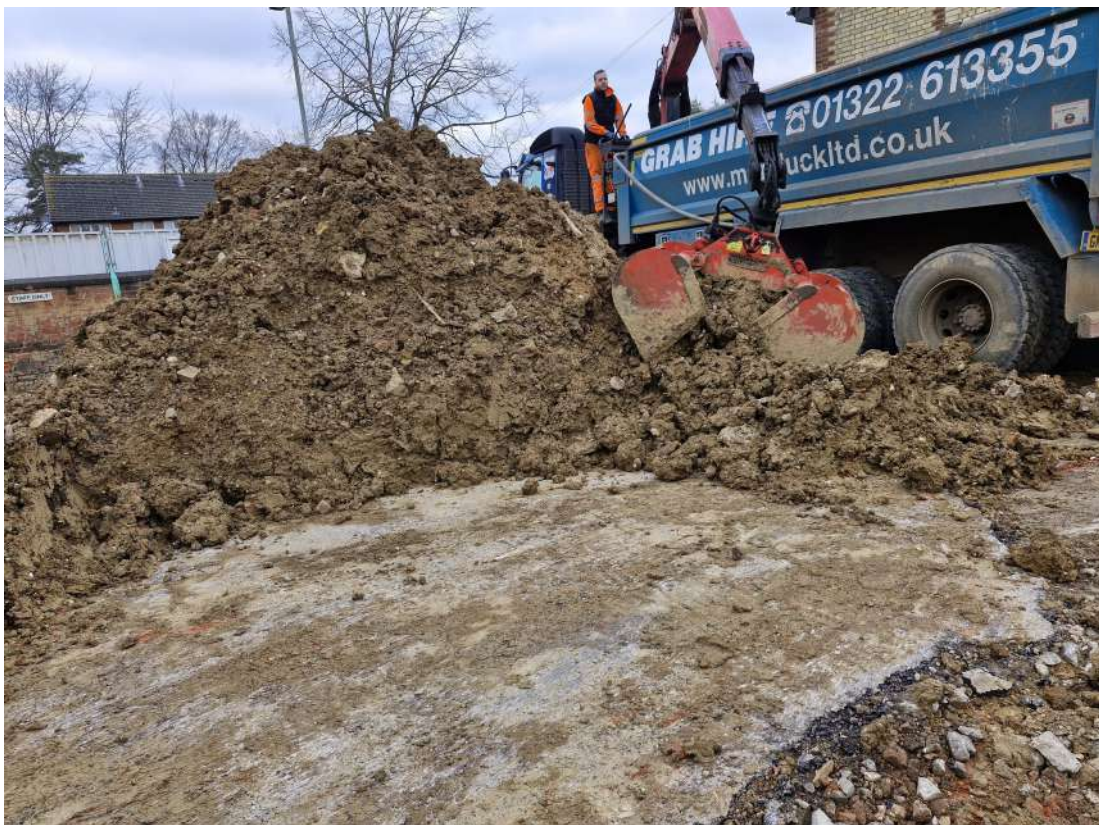
Photo 2: Showing the removal of Non-Hazardous waste.
