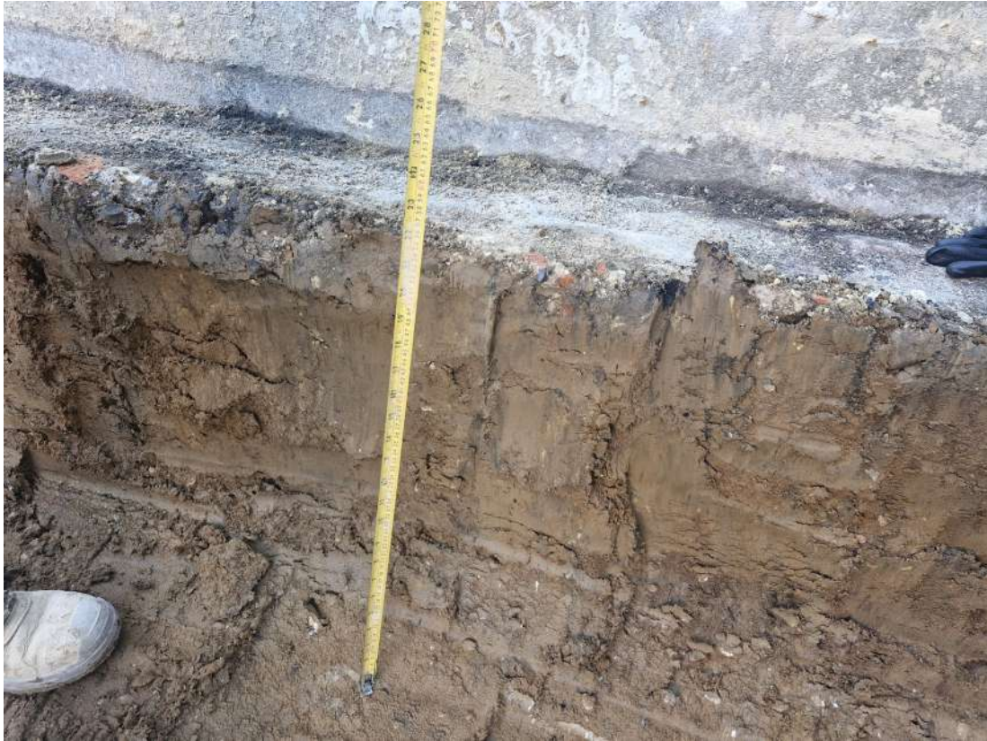
Photo 3: Showing the Remedial excavation of the contaminated hotspot to the required depth.
