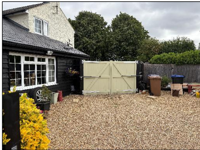
Photograph 5 Driveway to east of site
