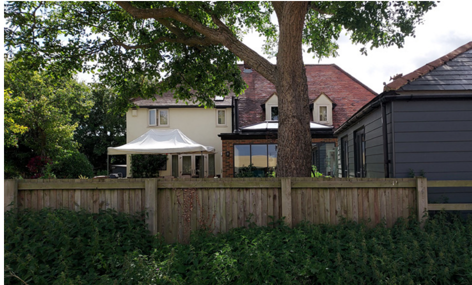
2. Greenleas Site - Rear view
