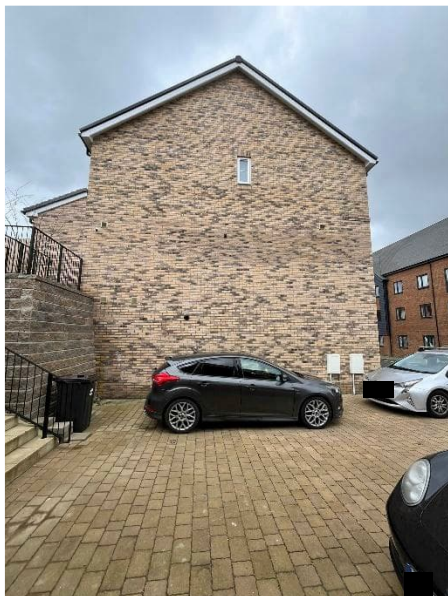
Image 2: Side elevation of the applicant's house
