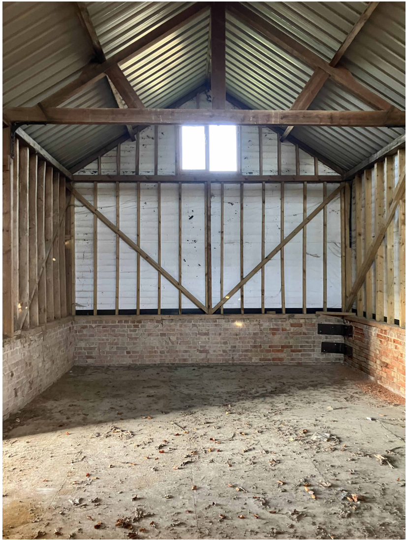
Roof truss
