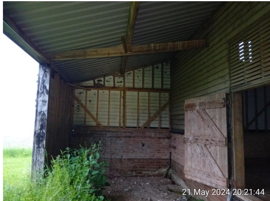
Figure 5: Example of interior.
