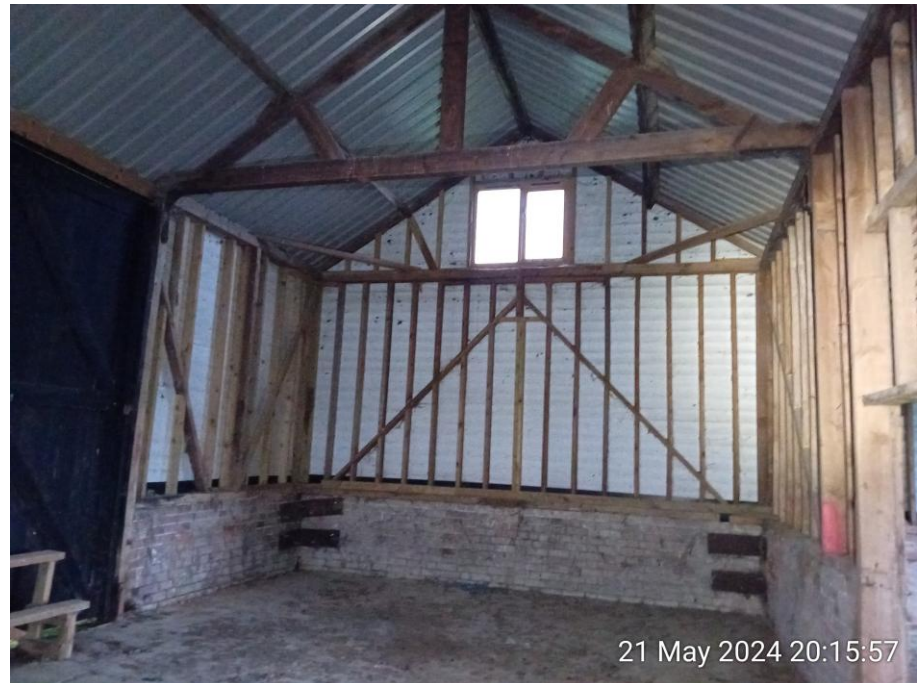
Figure 4: Example of interior.
