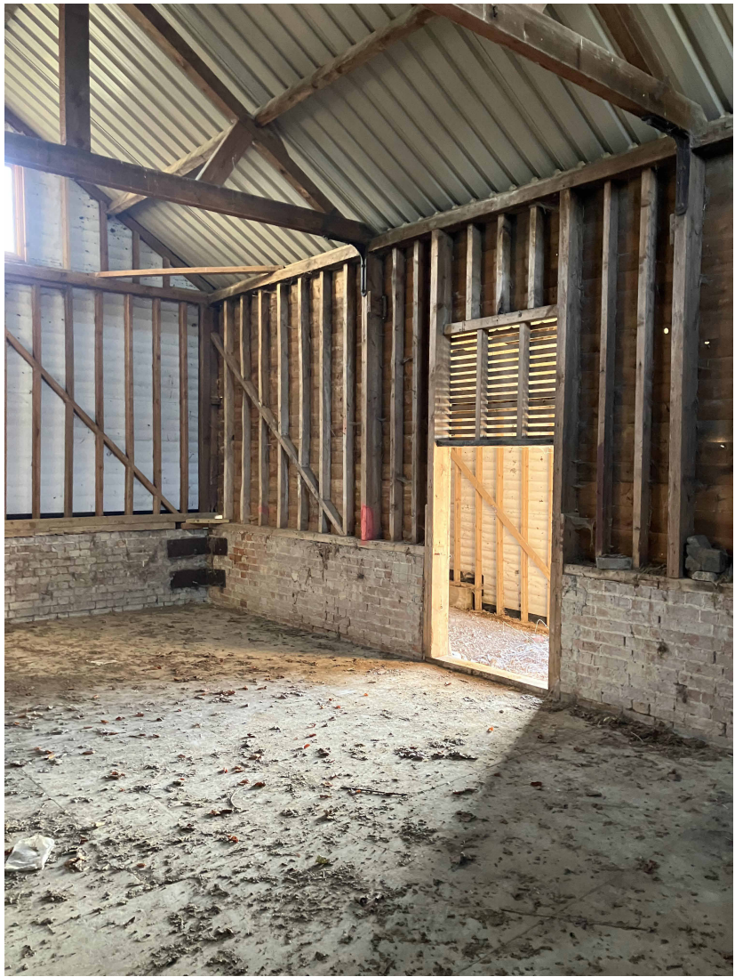
Internal feature wall
