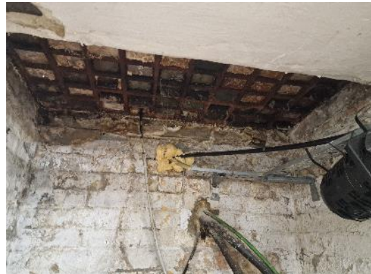
Photograph L – Pavement light
