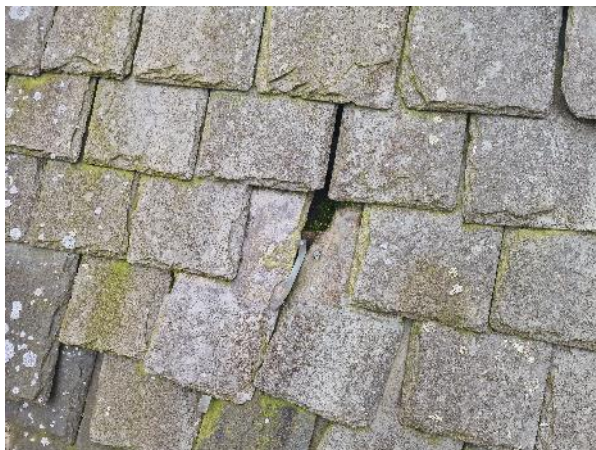
9. Damaged slates
