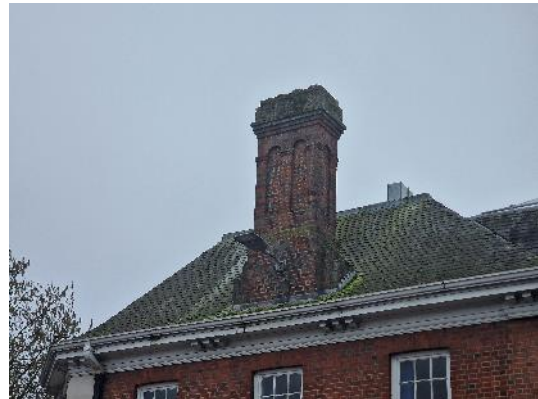
Photograph H – Chimneystack
