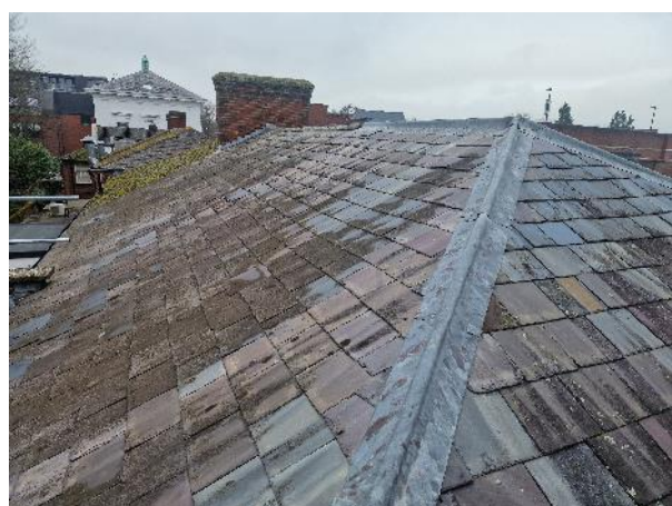
6. Roof to rear projection
