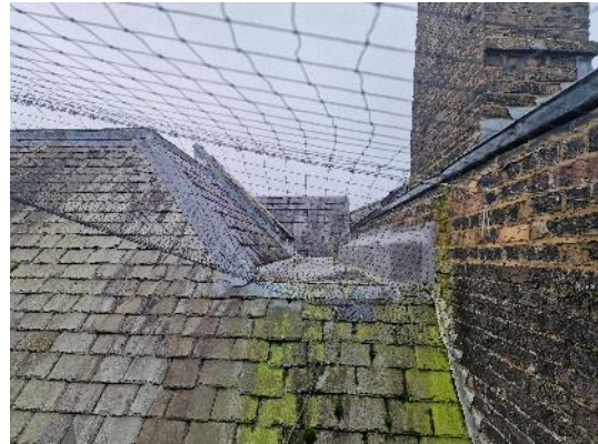
Photograph B – Channel gutter
