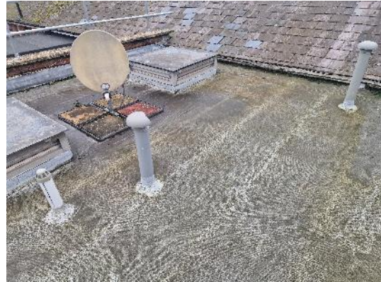
Photograph E – Lower flat roof
