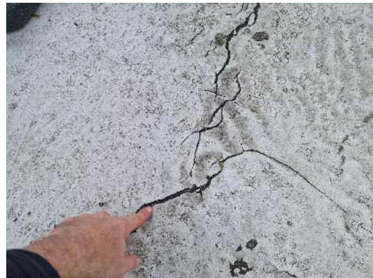
Photograph A – Cracking to asphalt
