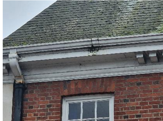
Photograph G – Rainwater goods
