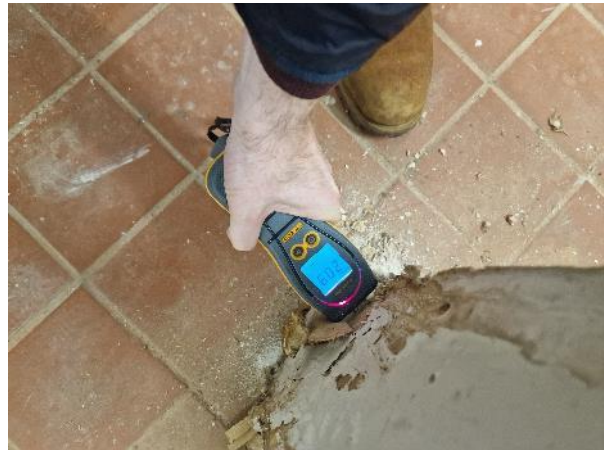
22. Timber decay to supporting post
