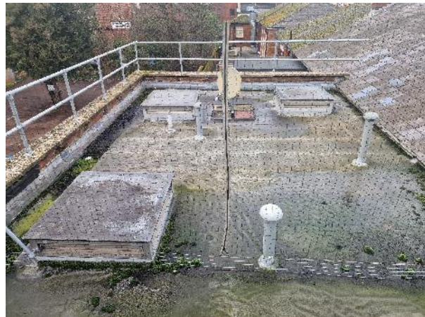
8. Flat roof to rear
