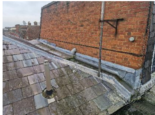
Photograph C – Pitched roof and valley
