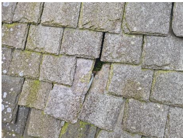
9. Damaged slates
