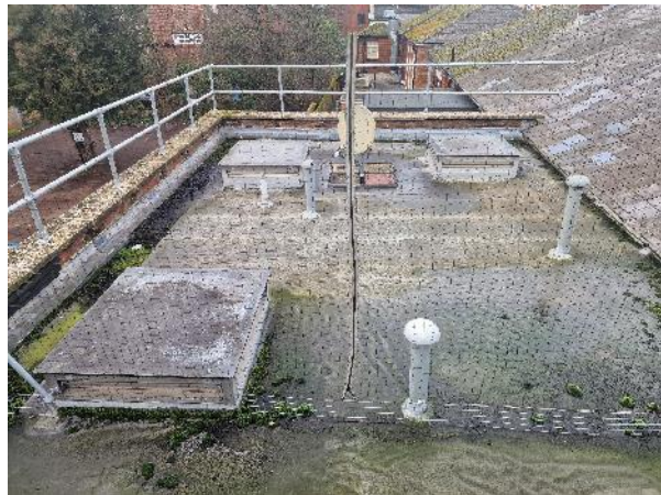
8. Flat roof to rear
