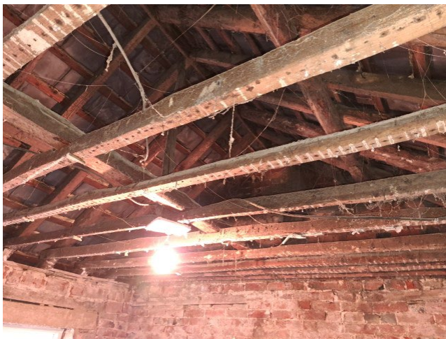
Photo 16 – View of the attic space
