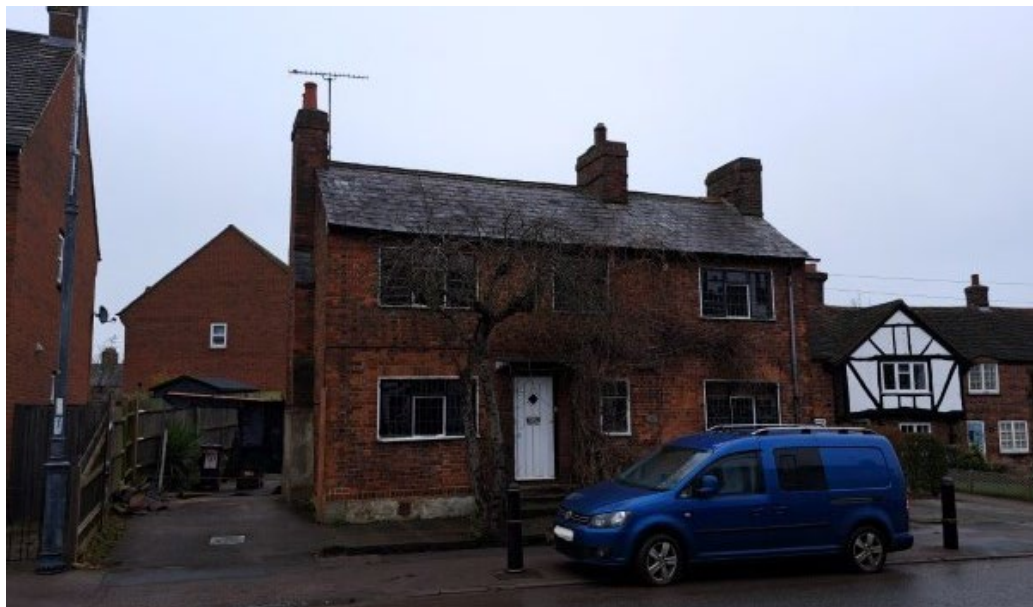
Photo 1 – View of front (south) elevation
