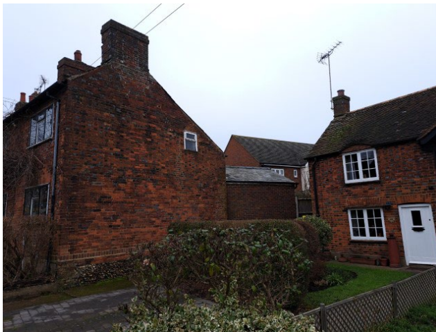
Photo 4 – View of the side (east) elevation
