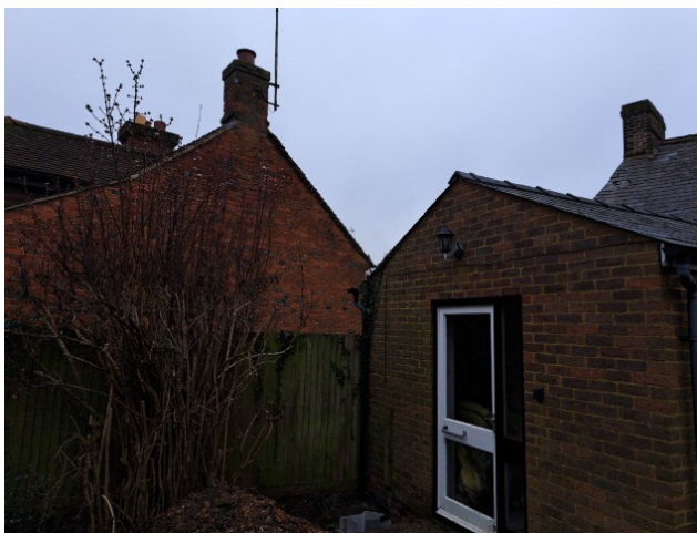
Photo 7-11 – View of the rear elevation and the existing extension
