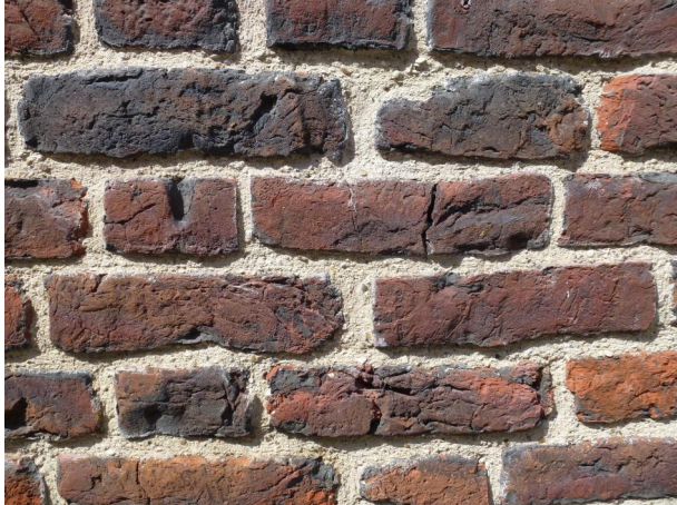
External Facing Bricks
