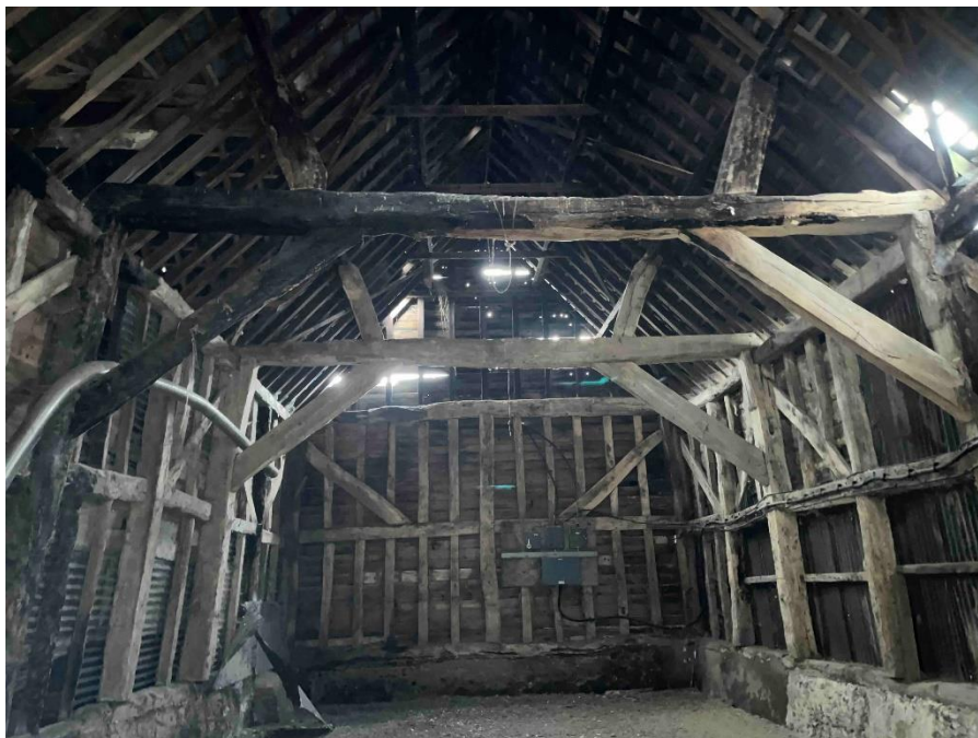
Image 1- Barn 1 internal view
