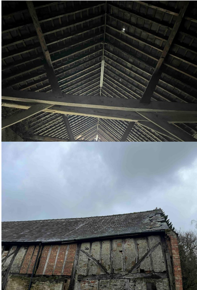
Image 2- Barn 2 internal and external view
