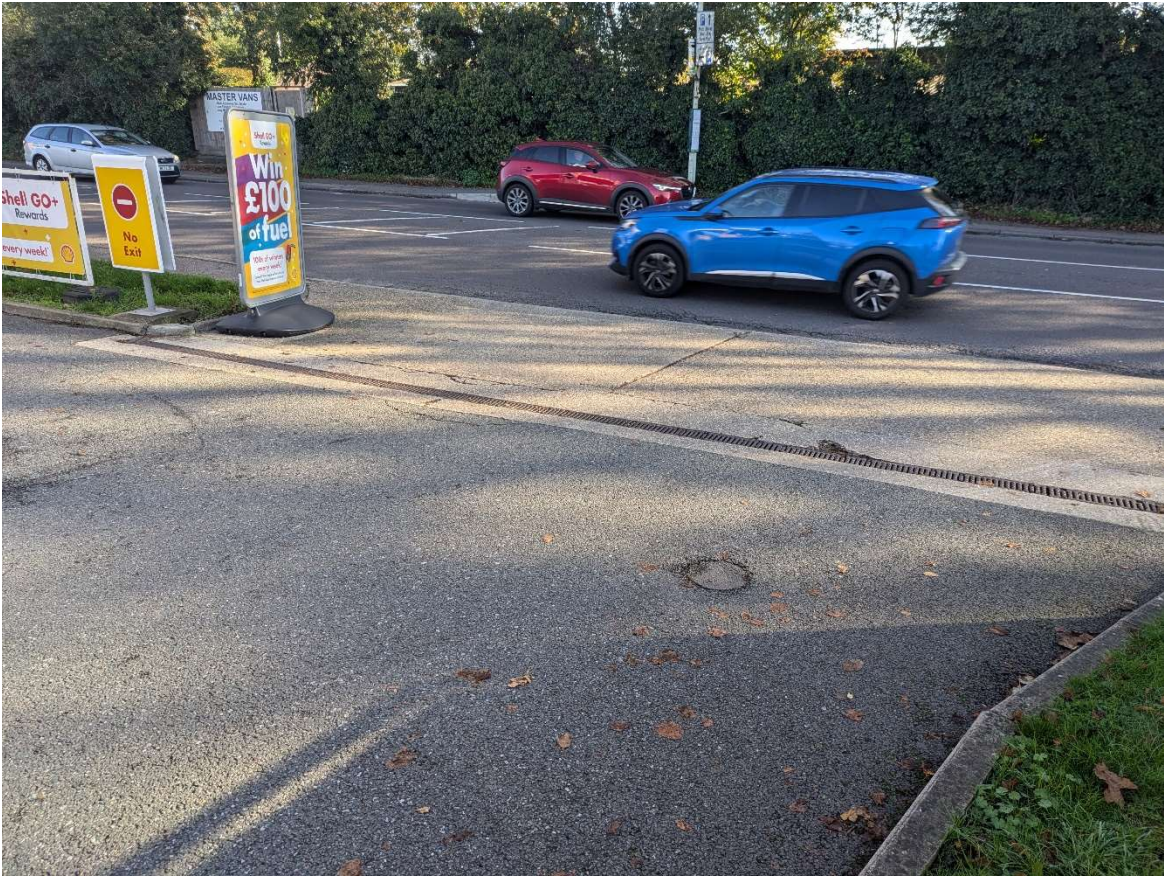
Evidence of previous boreholes identified near the southeast region of the Site
