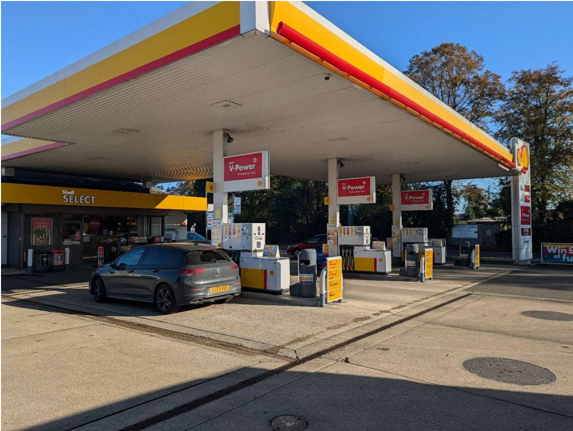
Shell Hitchin Forecourt facing southeast
