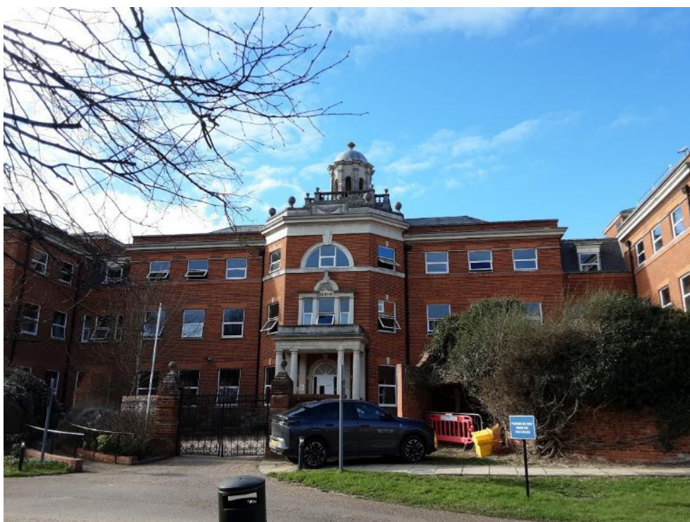
Photograph 6: Radcliffe House (UB1).
