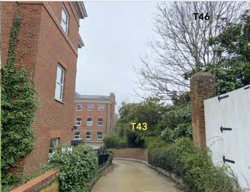
IMAGE 5: View of the existing access ramp and retaining wall at the northern access from Old Charlton Road, looking southwest.
