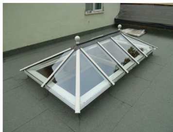
EXAMPLE Traditional timber roof lantern
