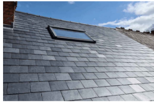
EXAMPLE OF SLATES TO MATCH EXISTING
