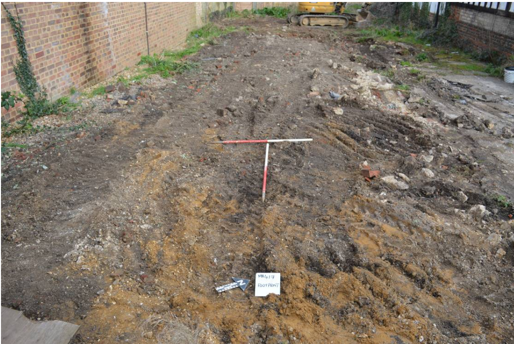
Plate 4: Made Ground Below Hardstanding – Looking North-West.
