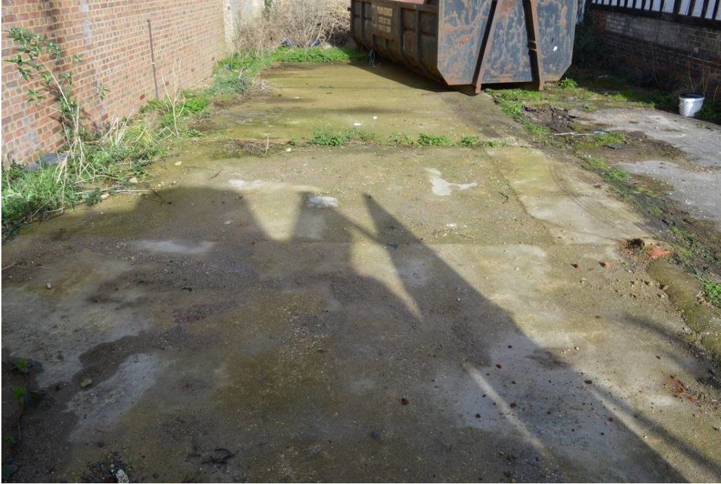
Plate 3: Concrete Hardstanding – Looking North-West.
