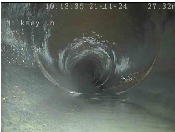
29270812-47d4-47e3-94d8-0189b74d66e6.png, 00:01:50, 28.00 m Roots, fine at joint
