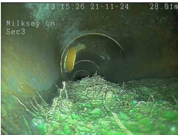
17d09909-7178-4815-81a0-ae1a1d9967ac.png, 00:03:26, 28.10 m Roots, mass, 40% cross-sectional area loss, change
