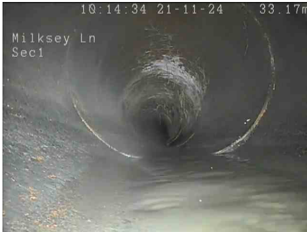
93e7a674-413d-43cd-a0ed-10f057f7ce26.png, 00:02:48, 33.50 m Roots, fine at joint, finish
