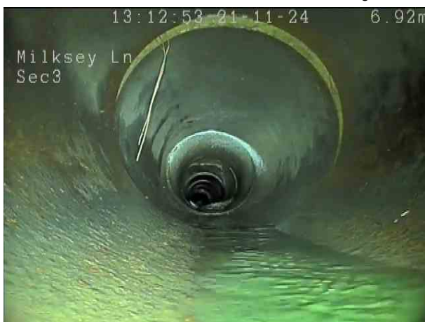
185b37ec-0349-4d34-8897-50f622d61a30.png, 00:00:53, 7.40 m Roots, fine at joint
