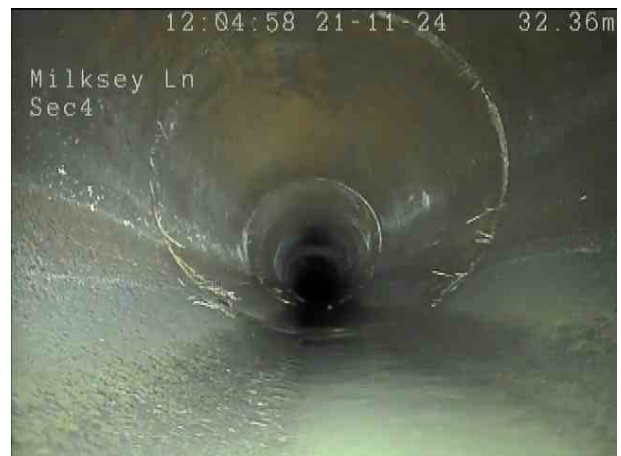
ced64048-de0d-4066-a821-b95732ef483e.png, 00:02:35, 32.80 m Roots, fine at joint
