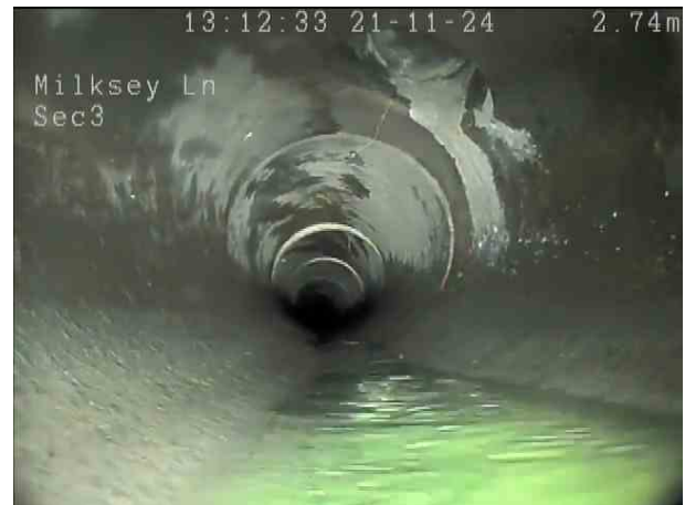
401ab29a-4c70-4d57-8003-c0800992f88c.png, 00:00:33, 3.10 m Junction at 1 o'clock, 150mm dia
