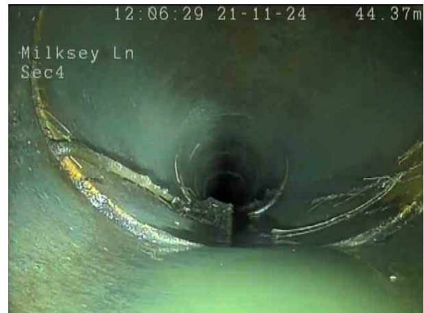
e6347e56-5449-4c1b-87a2-0c68d97f732a.png, 00:03:57, 44.50 m Roots, tap at joint, start
