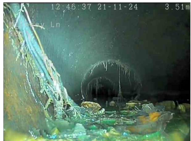
03c760a4-c011-424d-a0e7-884292924b45.png, 00:00:35, 3.50 m Roots, mass at joint, 30% cross-sectional area loss, change
