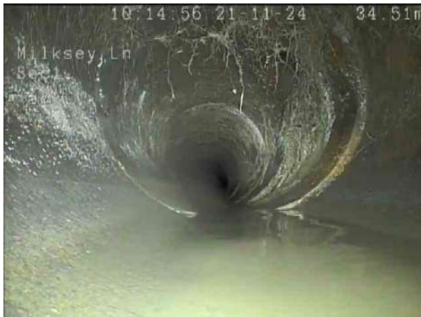
f539d5c1-cff1-4d3c-b9ef-aa45644b736d.png, 00:03:10, 35.00 m Junction at 2 o'clock, 250mm dia
