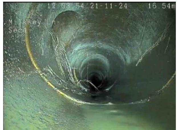
777f24de-9b4a-467c-a4c1-97b24560e6a4.png, 00:01:31, 16.90 m Junction at 10 o'clock, 150mm dia
