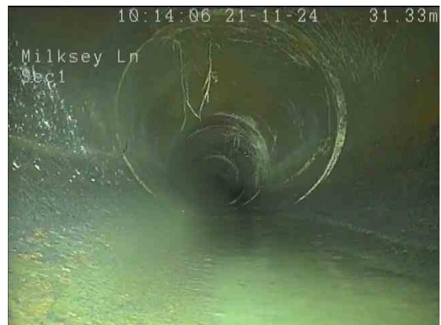
f2520338-991b-4d49-a4b7-b083027ddd3.png, 00:02:21, 32.00 m Roots, fine at joint, start
