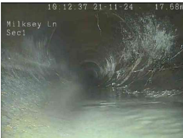
b2a526c9-151c-40f6-809e-3401277c87f8.png, 00:00:51, 18.20 m Roots, fine at joint, start
