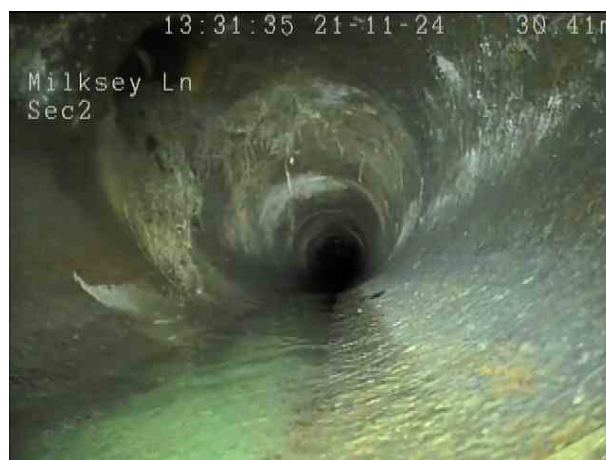
a02fb6f8-db22-495e-b60a-9fe1844e9d07.png, 00:02:32, 31.00 m Junction at 10 o'clock, 150mm dia
