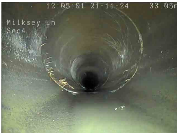
bafb911b-6cbc-4a8f-9351-8adddeb6f59d.png, 00:02:38, 33.50 m Roots, fine at joint
