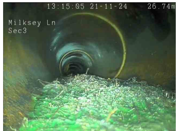
834ecfe2-25ef-439e-99da-13f364f33e35.png, 00:03:05, 26.80 m Roots, mass, 20% cross-sectional area loss, change
