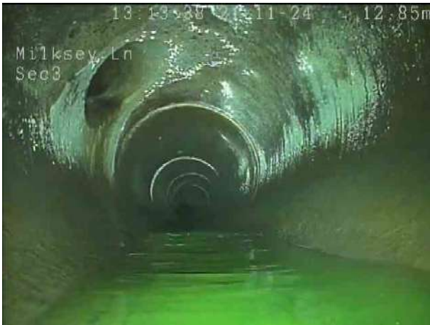
ced530b9-5c45-4fb0-bd8a-c44cf9934782.png, 00:01:38, 13.20 m Junction at 10 o'clock, 150mm dia
