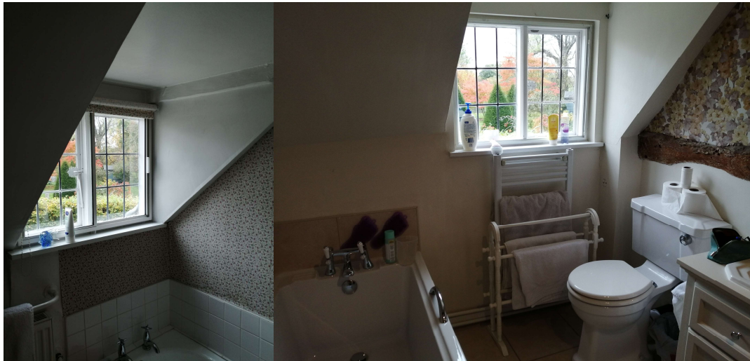
Left: Existing bathroom (Righthand side wall being removed) Right: Existing bathroom (Lefthand side wall being removed)
