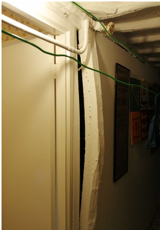
Link corridor with 'wonky' post to side of existing modern opening in wall.
