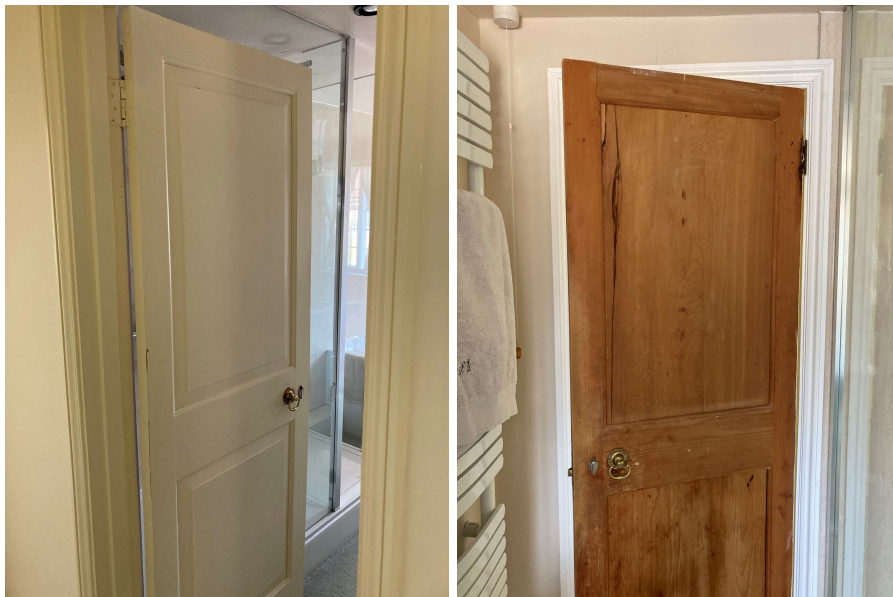
Existing door into Master Ensuite from corridor side and bathroom side
