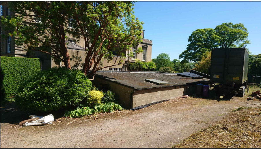
Photograph of Rear of Service Building
