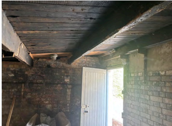
Image 6 - Interior of west portion of B1.
