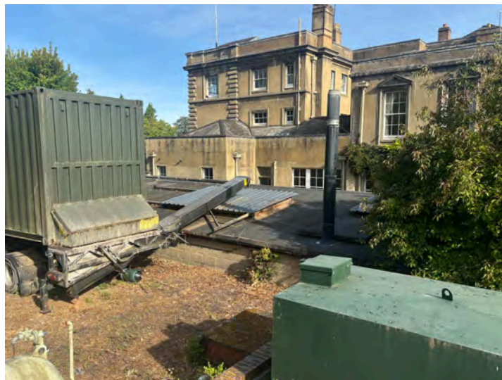
Image 4 - Roof and equipment to the south of B1.
