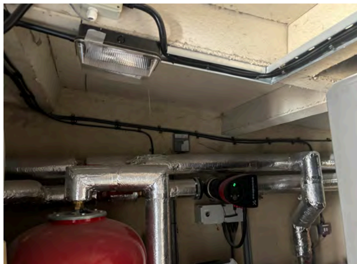
Image 8 - Interior of eastern/central portion of B1.
