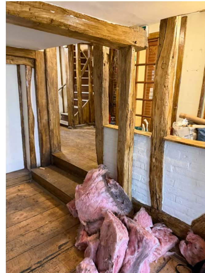
As Existing - Room side
