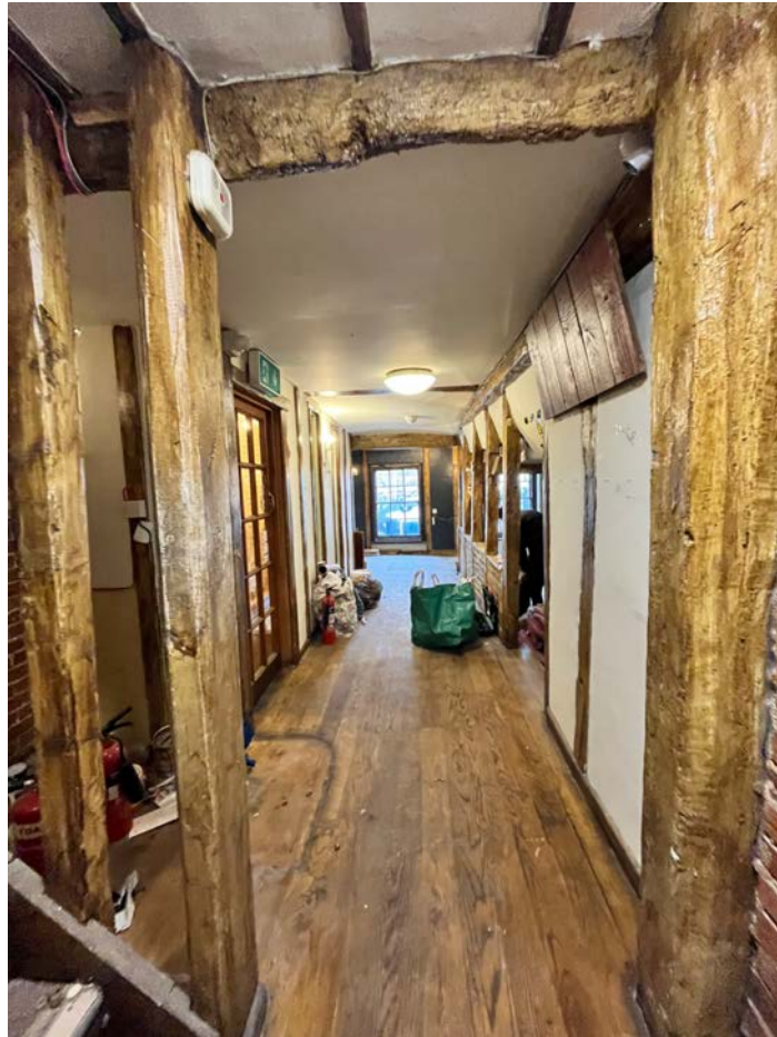
As Existing - Hallway
