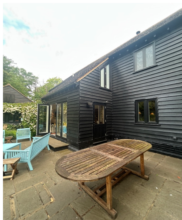
North dining room openings
