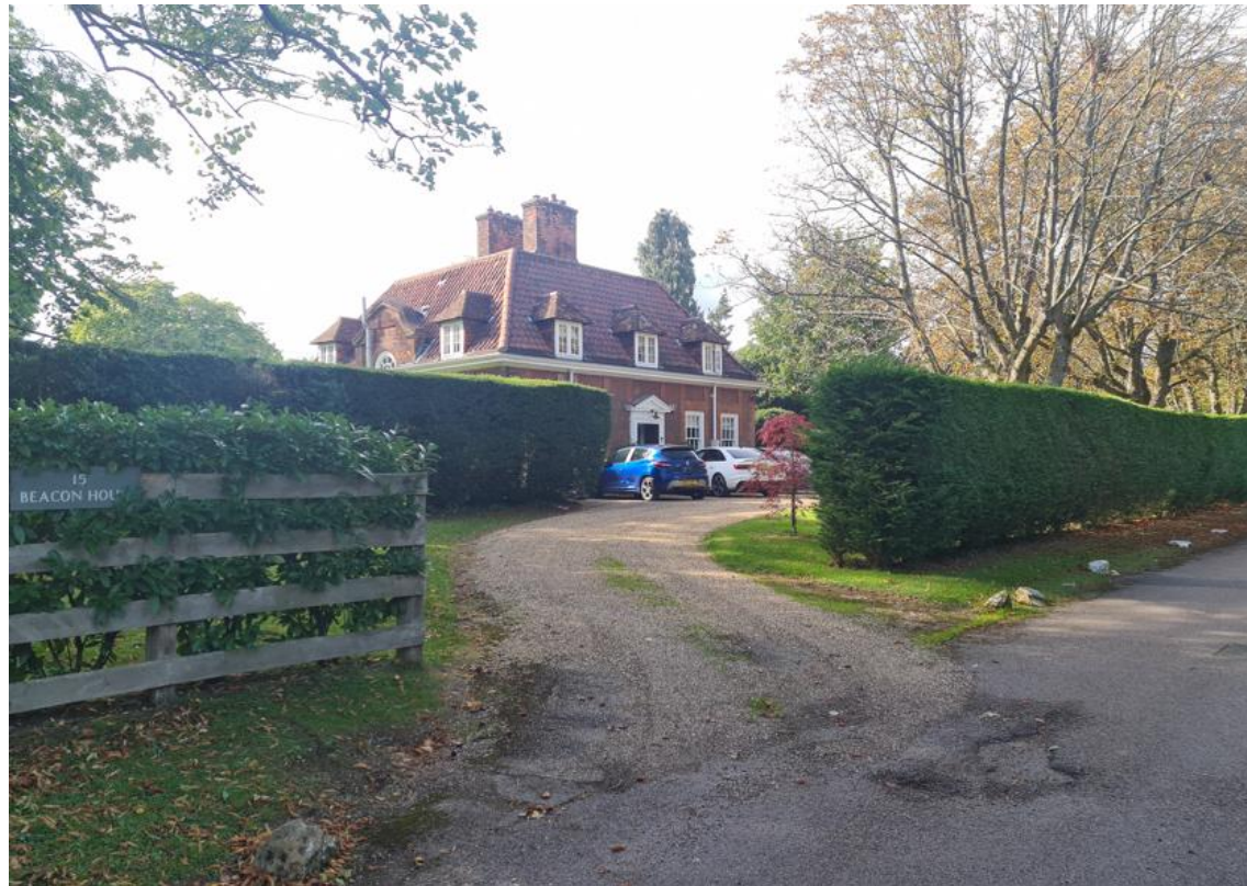
Figure 3 – Southern access to 15 Deards End Lane
