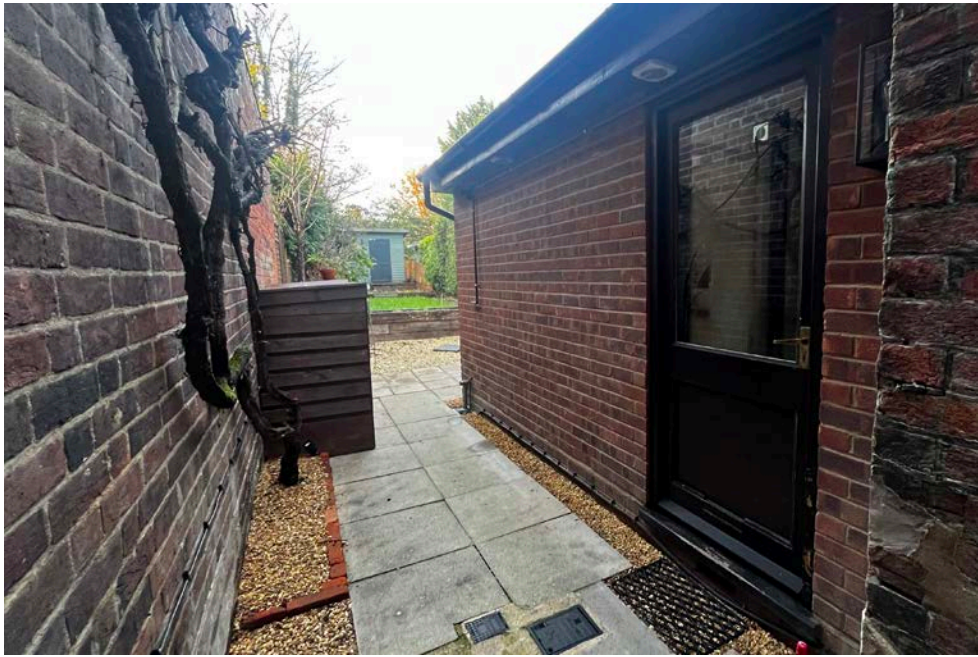
Existing rear extension/side
